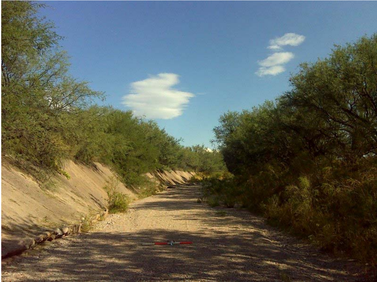
Figure 1. Straightened Reach of Sonoita Creek (looking upstream) with Concrete Armored Streambank (Courtesy of Westland Resources)
