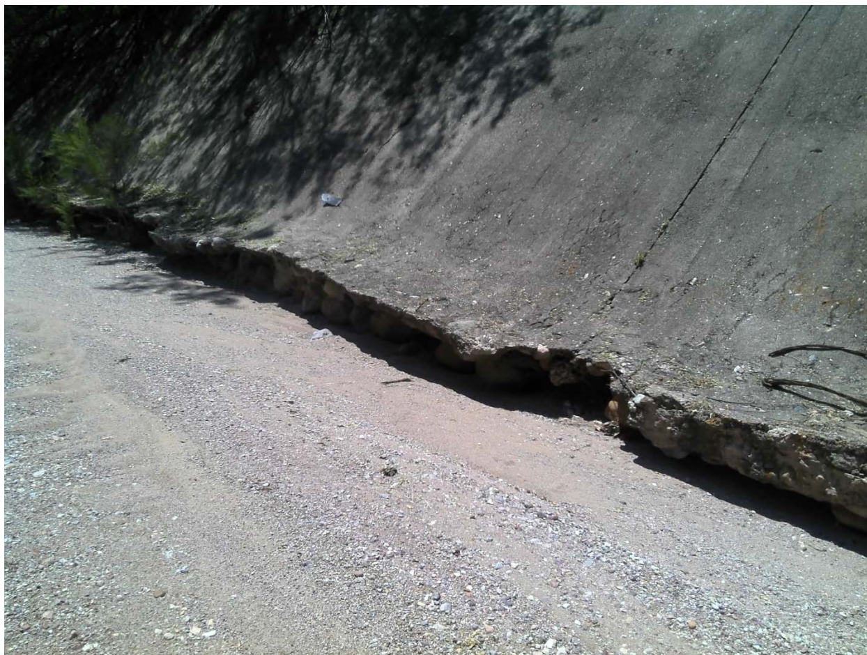
Figure 2. Sonoita Creek Armored Bank with Toe Scour and Limited Ecological Function (Courtesy of Westland Resources)
