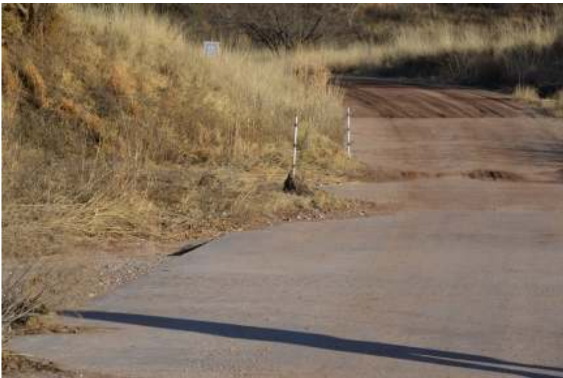
Figure 4. Road Crossing (Second of Two Photos; Downstream to the Right) with Visible High Water Marks and Debris Accumulations
