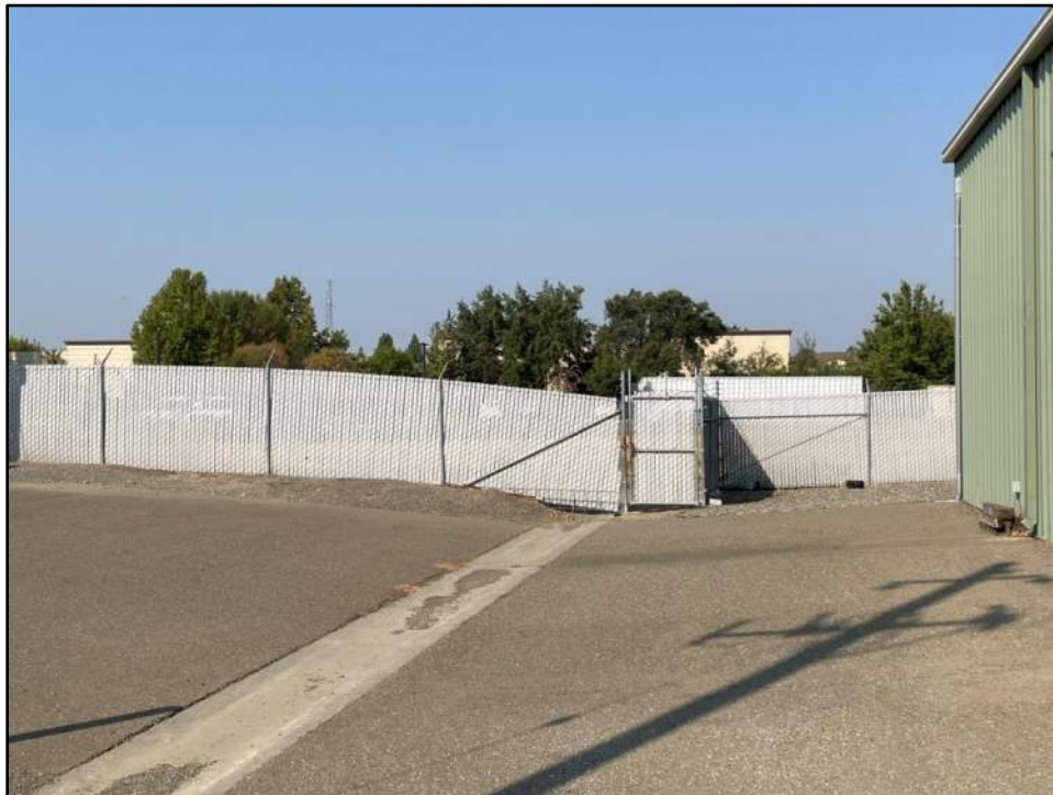
Photograph C-8: View of drainage leading into upland swale, facing west.
