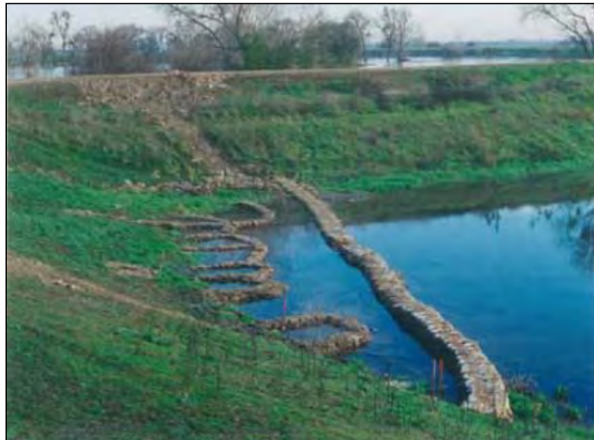
Figure 2-10: Seepage and Sack Rings 1997, RD-17 (≈RM 9.5)
