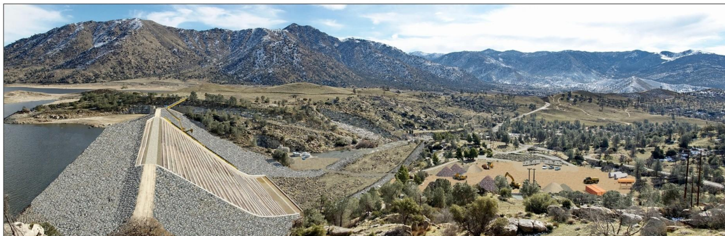
Simulation of Main Dam 800-ft RCC Overlay with Fuse Plug, Staging Area M1, portion of Emergency Spillway, and Concrete Conveyor. Alternative Plans 1, 2, and 3.
