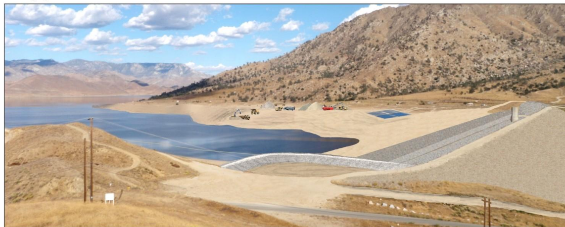
Simulation of Staging Area A1, Sand Borrow Site and Washing Area, Water Holding Ponds, Haul Roads H1 (foreground) and H5, and Cofferd Dam. Lake elevation at 2,543.76 feet (NAVD 88).
