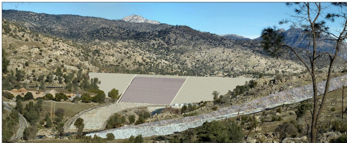
Simulation of Main Dam with 800-ft RCC Overlay and Fuse Plug, visible portions of Emergency Spillway, and Staging Area M1. Alternative Plan 2.
