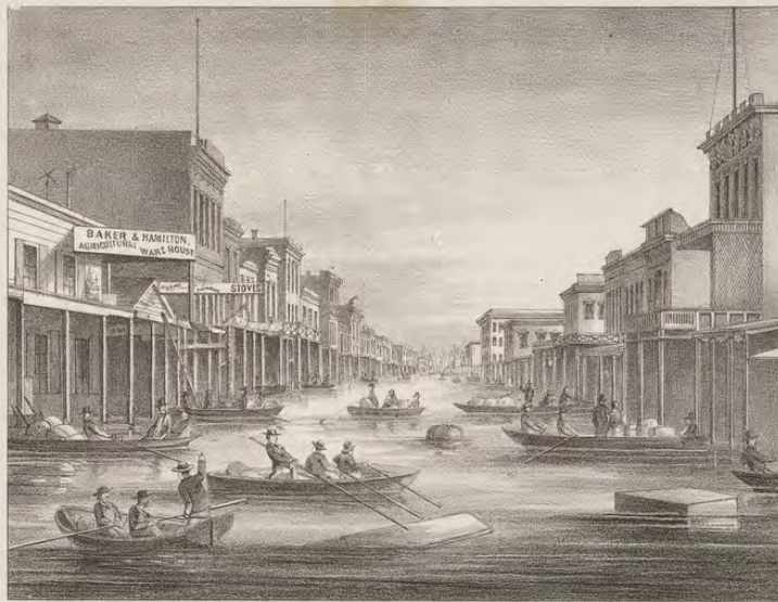
J. STREET, FROM THE LEVEE.
