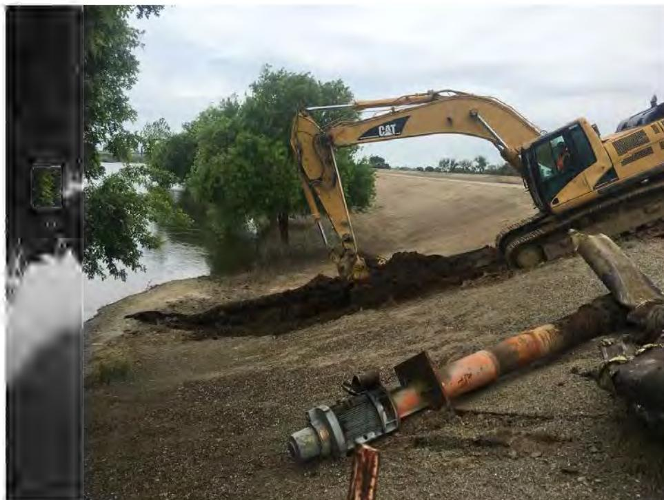
**Photograph 1.** Removal of water pipe crossing the levee before construction of the seepage berm.
