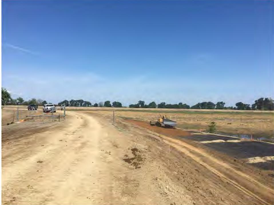
**Photograph 2.** Spreading topsoil over fabric, the fabric is intended to prevent mixing between the soil and gravel layers.
