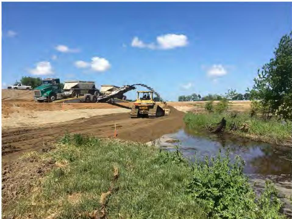
**Photograph 3.** Spreading sand at the base of the seepage berm within the project area to prevent erosion.
