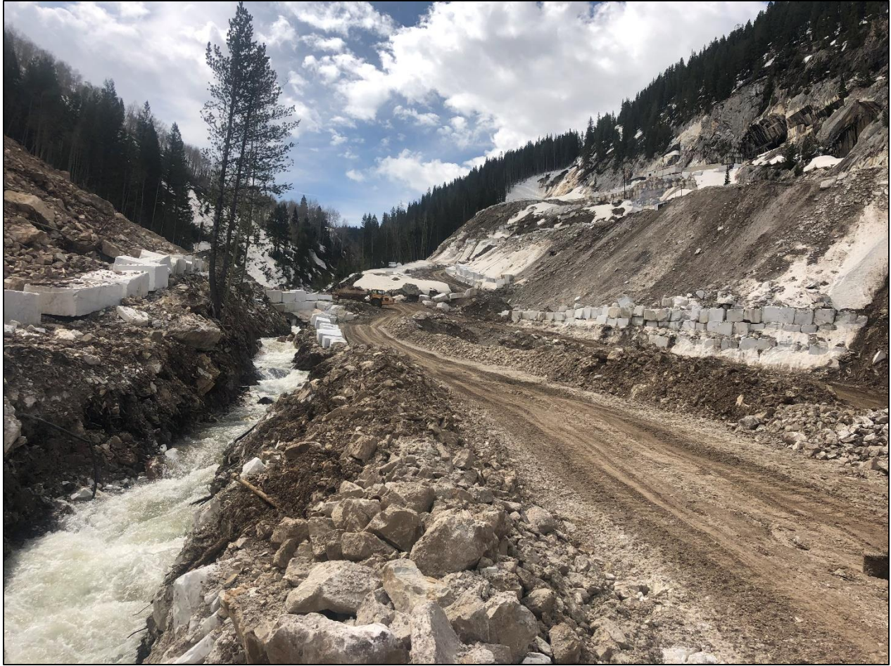
Figure 5: Off-highway vehicle and equipment access to the Franklin Quarry from the east adjacent to the eastern Yule Creek alignment along cross-section alignment 15+00. This area represents the area of the eastern alignment to be armored and widened as detailed in Alternative 2. The dump truck in view is parked adjacent to the diversion point. View to the south, photo captured May 5, 2019.
