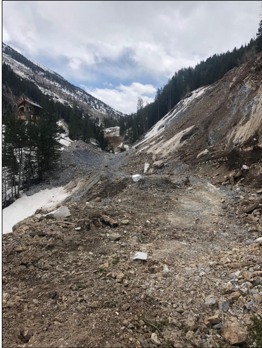
Figure 2. Post-blast smoothing of Belden shale at the northern extent of the access road along cross-section alignment 6+00. The small cabin on the Franklin Ridge is now removed and was located at cross-section alignment 9+00 (location of Figure 4). View to the south, photo captured May 15, 2019.
