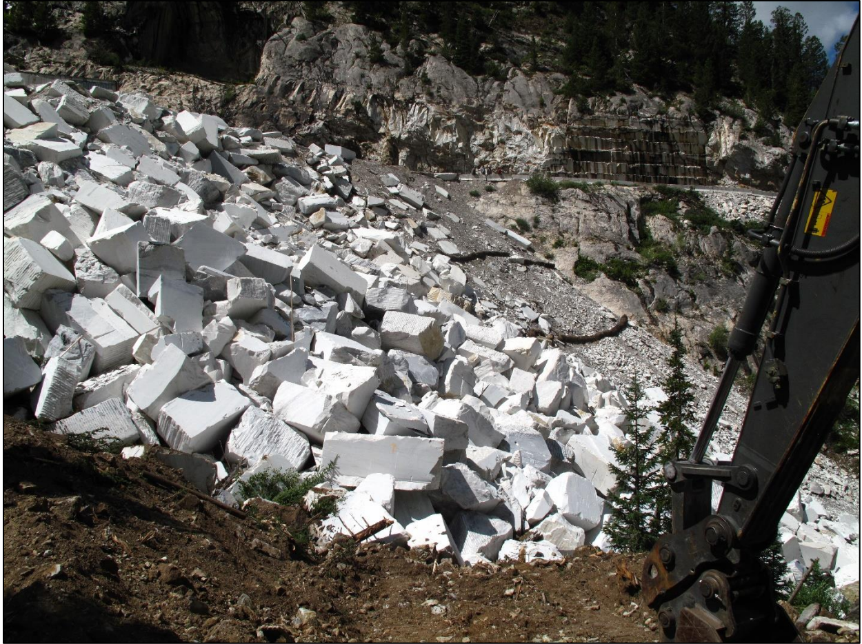
Figure 7: View of the upper Washington waste rock landform (dump) prior to the initiation of TR-05 construction along cross-section alignment 18+00. Marble rip-rap caps the 1.5H:1V slope above the marble block retaining wall. Notice the bedrock cliff to the west-northwest of the slope. View to the west, photo captured August 12, 2010.
