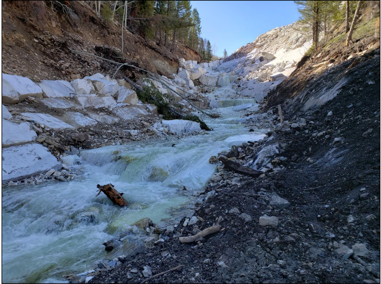
Figure 3: 2020 Erosion control structures (armoring) and velocity attenuators installed within the eastern channel along cross-section alignment 6+00. View to the south-southeast, photo captured May 13, 2020.
