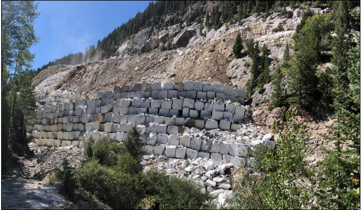
Figure 6: View of the Washington waste rock landform (dump) prior to the initiation of TR-05 construction along cross-section alignment 17+00. Marble blocks are stacked at a 0.5H:1V slope and abut the bedrock cliff to the west. The near vertical marble block wall is backfilled with mixed sized waste to create an unmovable and stable site derived waste management structure. View to the south-southwest, photo captured August 30, 2018.
