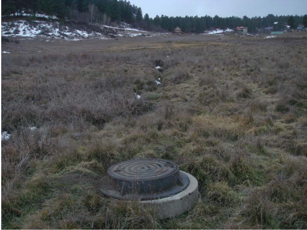
Photo Point 1. Looking southwest from Photo Point 1. Note existing sewer pipe parallels portion of channel. Channel varies from 1 to 3 feet deep and 1 to 3 feet wide.
