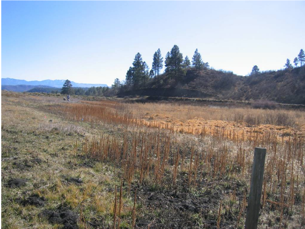
Photo point 1. Abandoned pond looking east across the breached dam.
