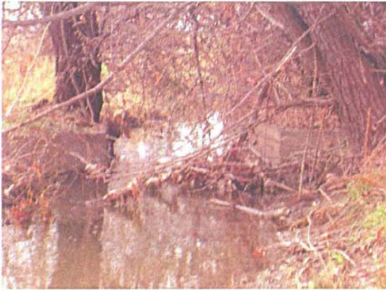
Photo 1. Shepard Creek. Irrigation structure on the creek, approximately 30 feet north of fence line.
