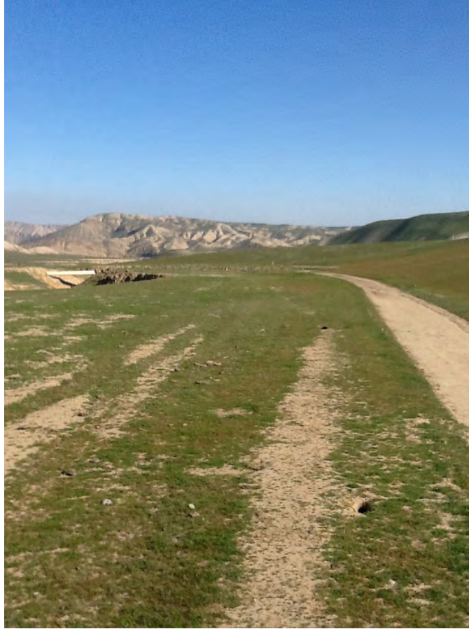
Figure 178: Photo 20b Facing east. Potential enhancement where drainage can be corrected and prevent drainage flow down the existing road and have water flow across
