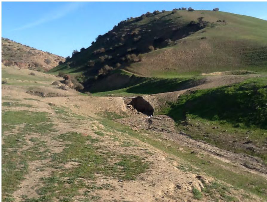
Figure 177: Photo 20a Downstream Old cattle dam possible removal for restoration. Four channels converge into primary, GIS does not show connectivity
