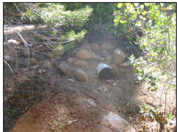
5d. – Culvert at ES-3 along Segment 4 of the Phase 2 trail alignment.
