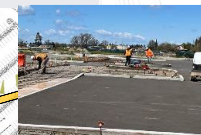
Installing Rebar North Side Parking Lot
