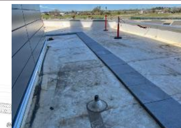
Concrete Pavers 2 nd Floor Roof
