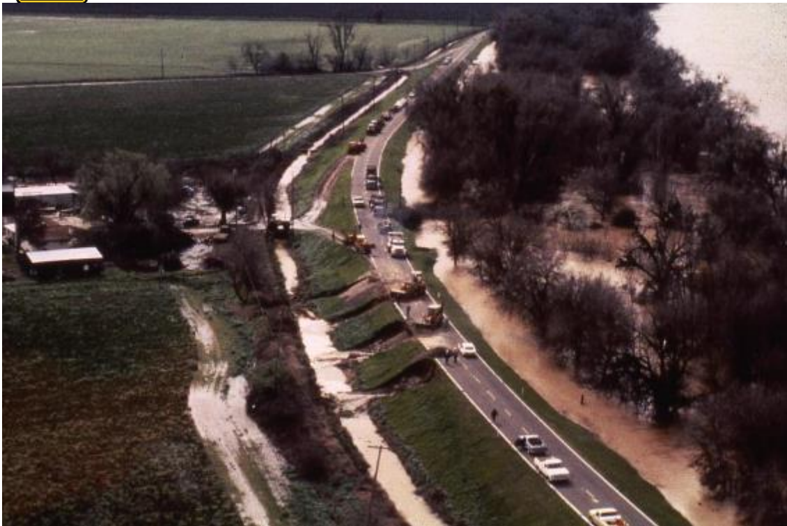
Levee land side levee sloughing caused by through levee seepage.
