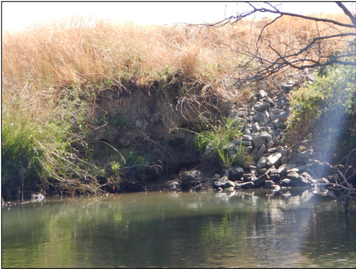
Figure 9. Erosion Pocket along the Georgiana Slough RM 4.5, Left Bank.
