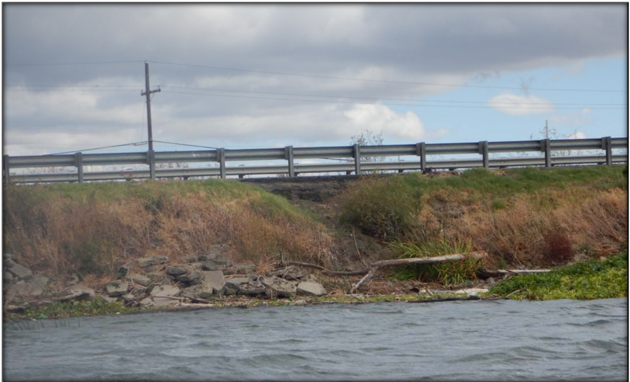
Figure 20. Erosion from Surface Runoff along the left bank of the Sacramento River at RM 7.9.
