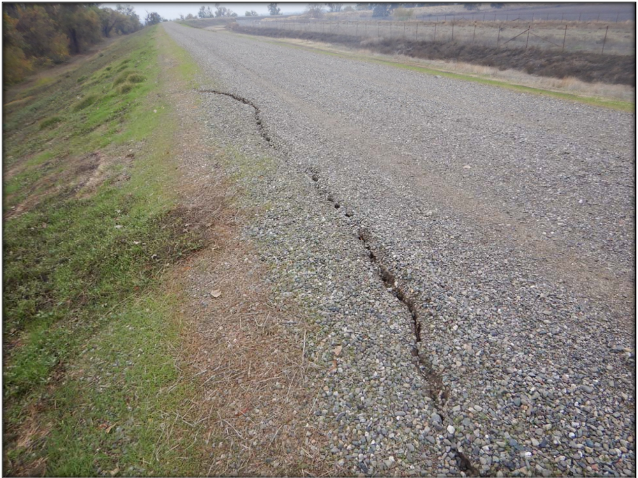
Figure 35. Slump Crack along the right bank of the Sacramento Bypass at LM 1.4.
