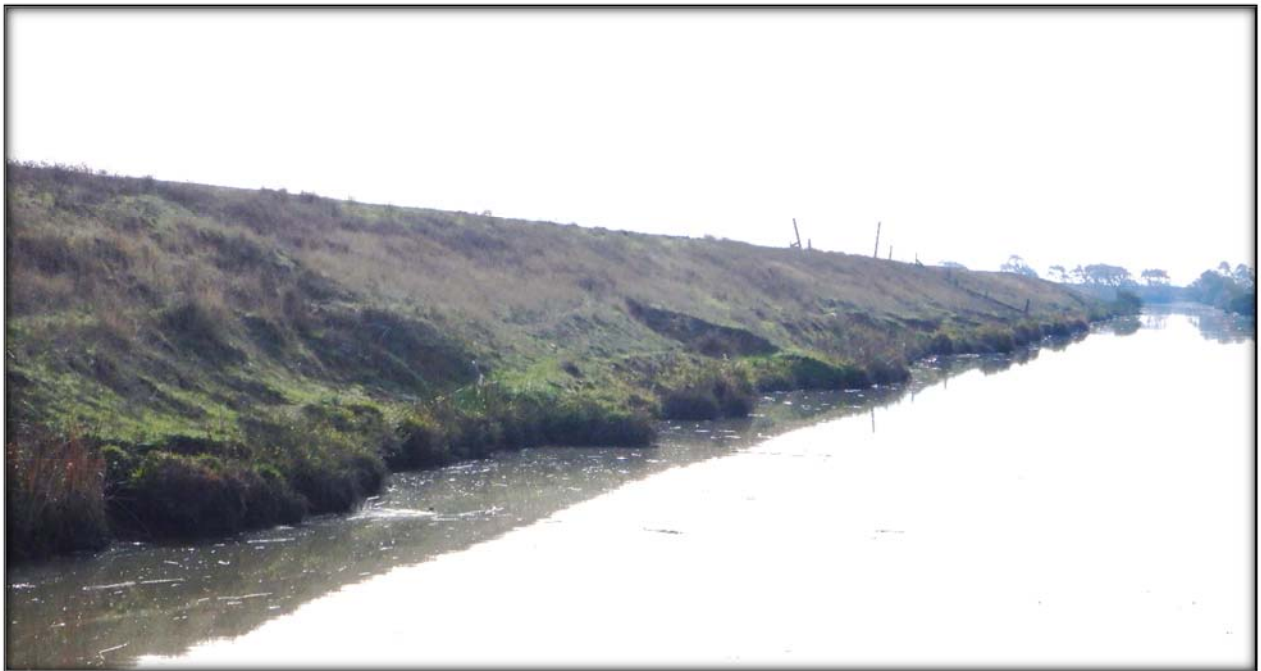
Figure 15. Erosion Pockets along the Left Bank of Haas Slough at LM 9.7.
