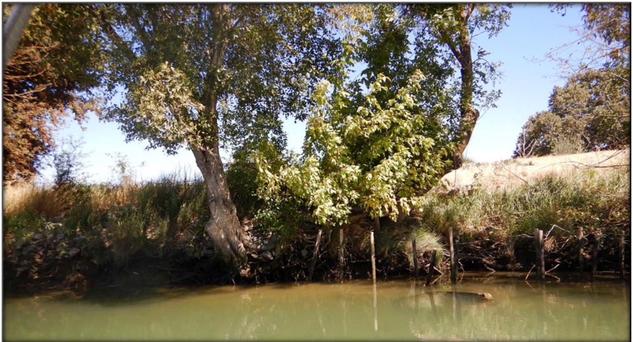
Figure 13. Photo depicting failing revetment and eminent tree pop-out at Georgiana Slough, RM 9.3L.
