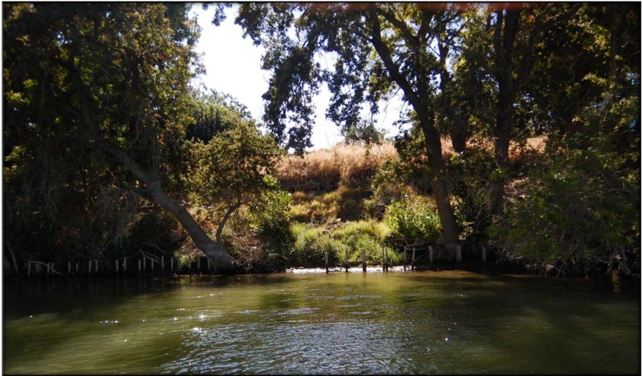
Figure 31. Toe scour and erosion of the levee slope along the right bank of the Sacramento River at RM 41.9. Empty brush boxes and leaning trees are also seen.
