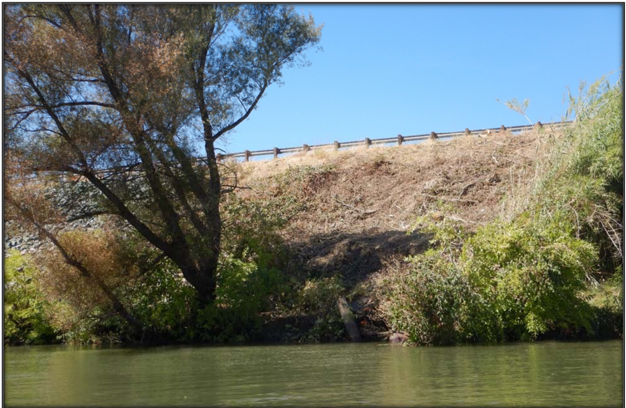
Figure 33. Eroded and over-steepened slope of the right bank of the Sacramento River at RM 55.7.
