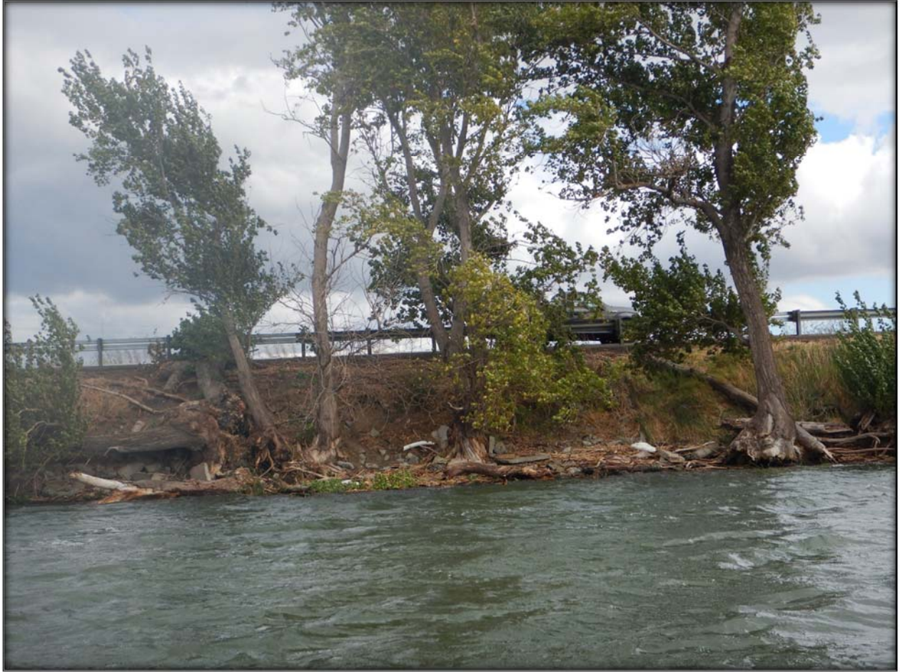
Figure 21 – Eroded levee slope and trees with exposed roots along the left bank of the Sacramento River at RM 7.9.
