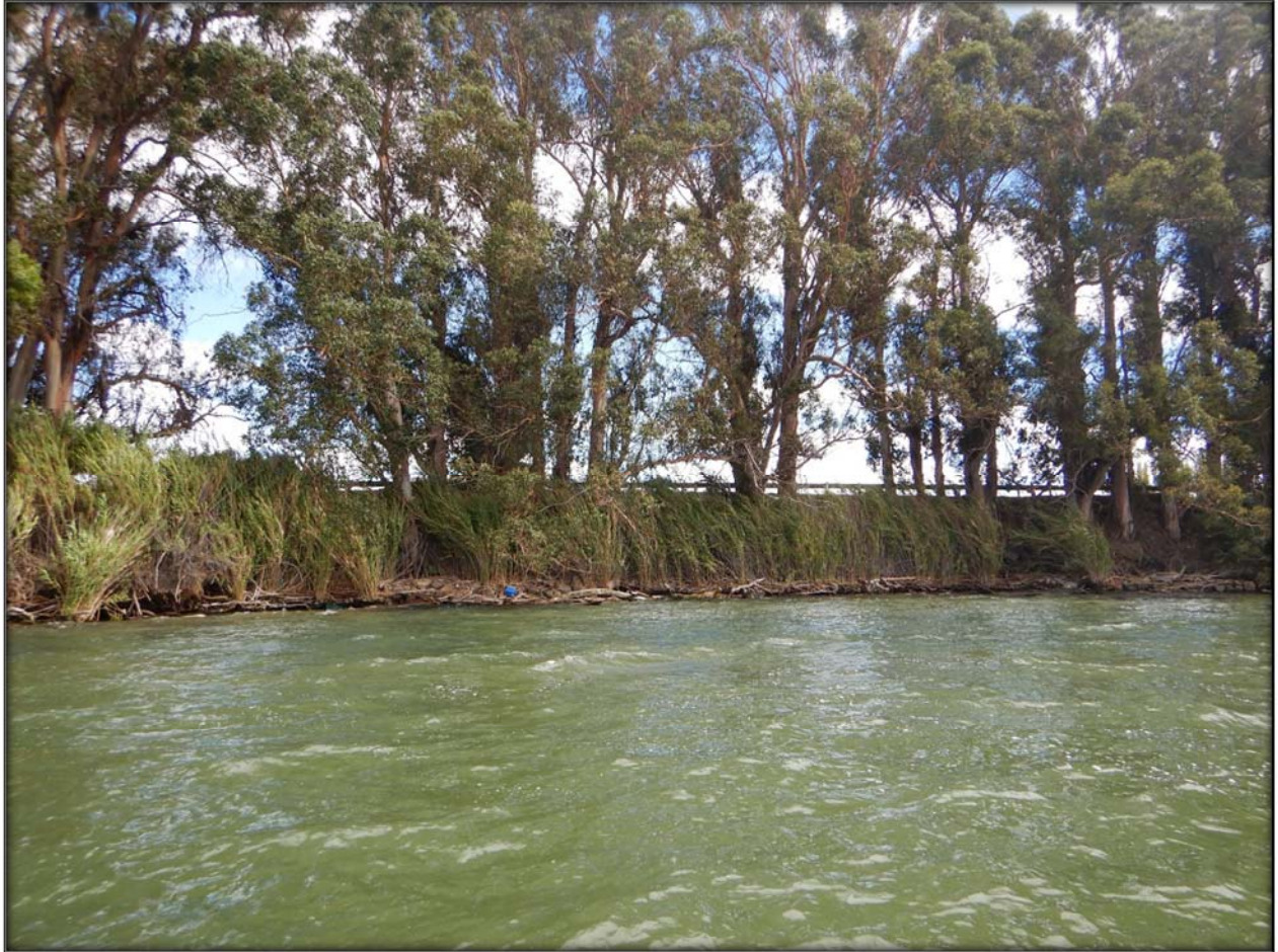
Figure 26. Eroded bank with large trees in the slope along the left bank of the Sacramento River at RM 12.1.
