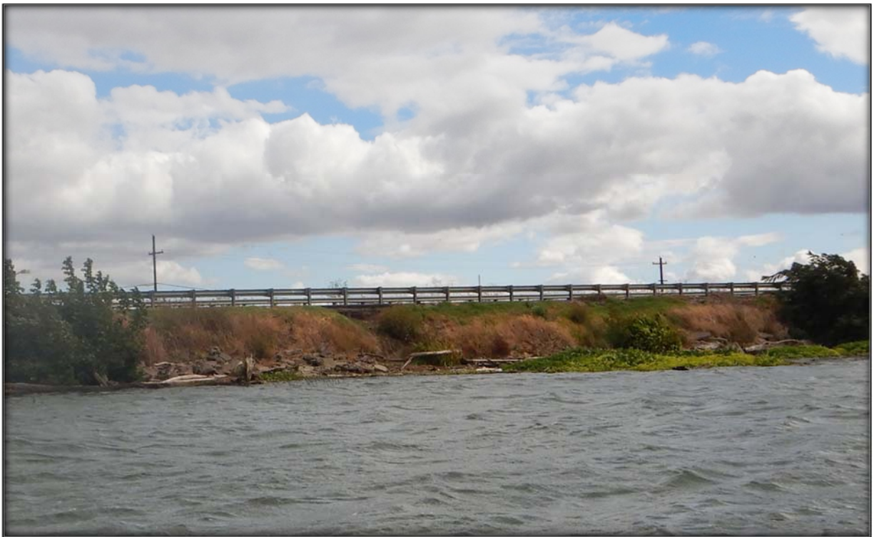
Figure 23. Erosion from surface runoff along the left bank of the Sacramento River at RM 8.0.
