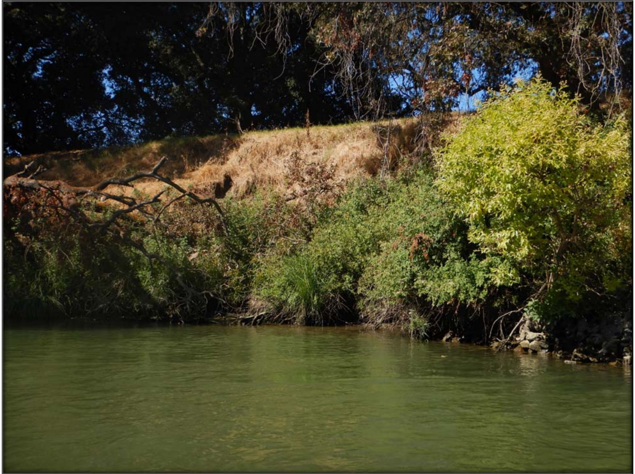
Figure 39. Eroding bank along the right bank of Steamboat Slough at RM 25.8.
