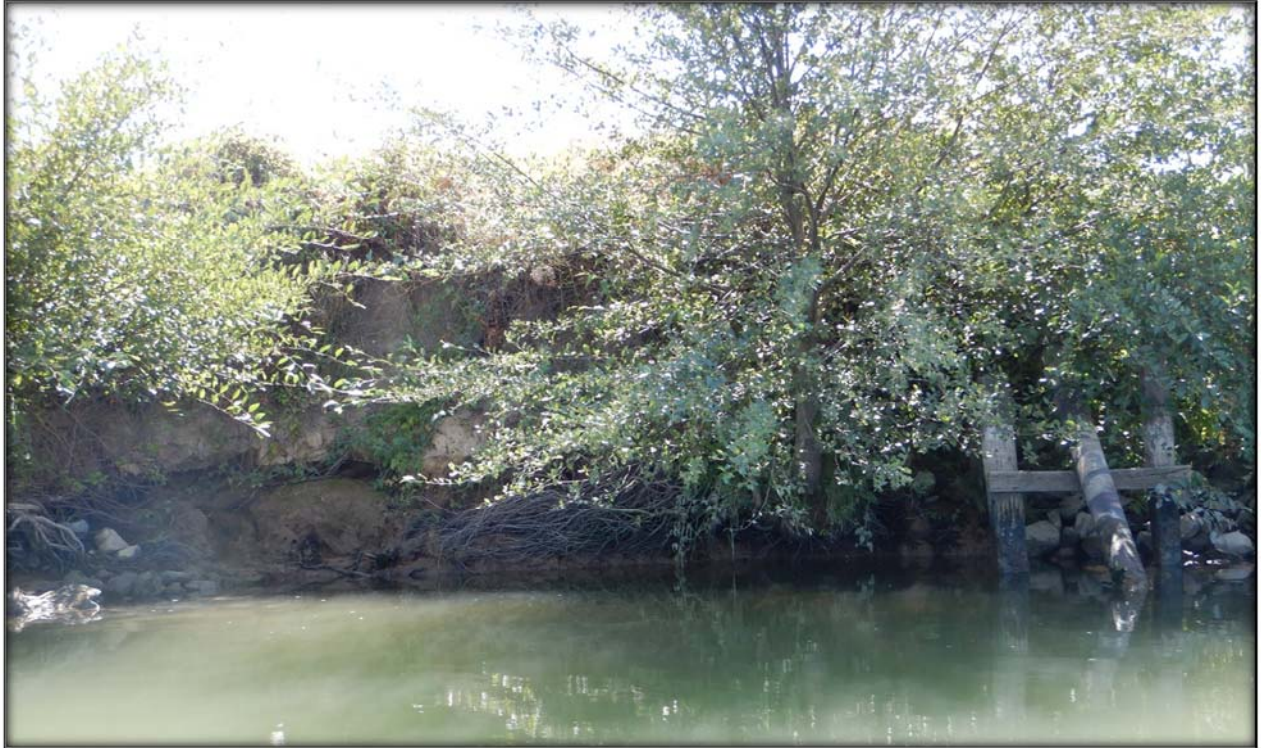
Figure 11. Erosion Pocket showing whole bank failure along the Georgiana Slough RM 6.3, Left Bank.
