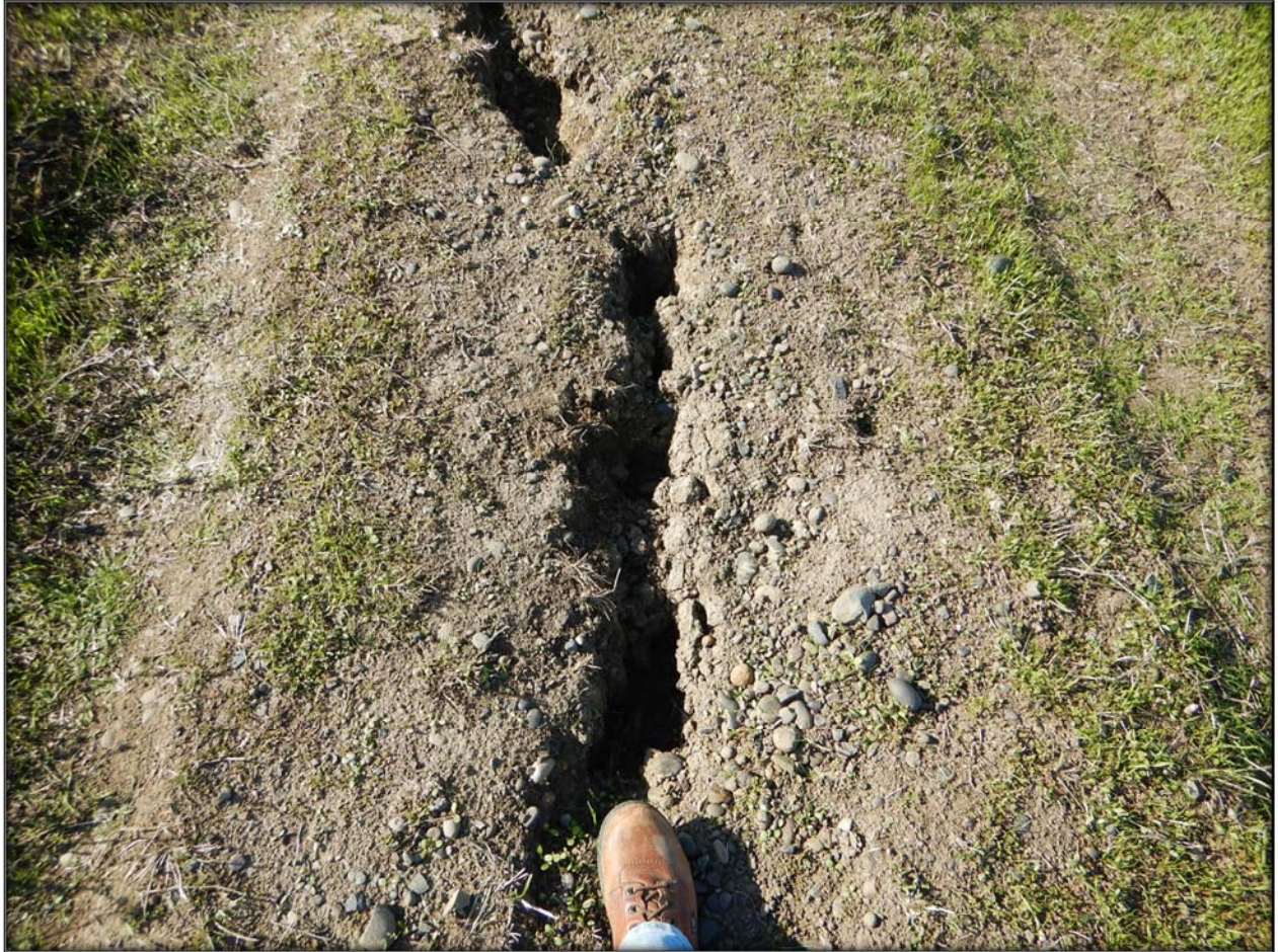
Figure 5. Slump Crack showing width of the crack (with boot for scale) at Cache Slough, RM 1.8L.
