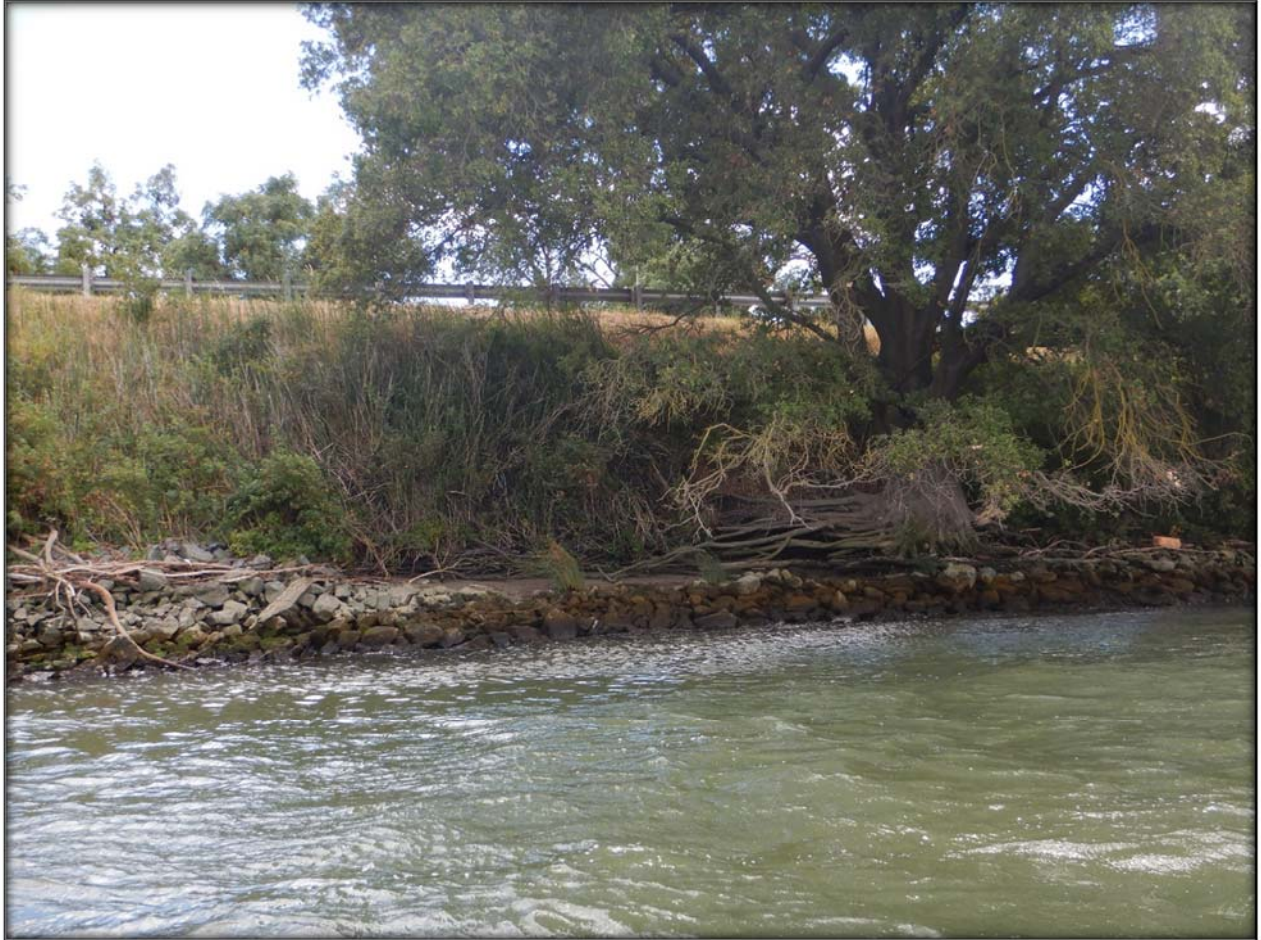
Figure 28. Eroded bank slope along the left bank of the Sacramento River at RM 18.1.
