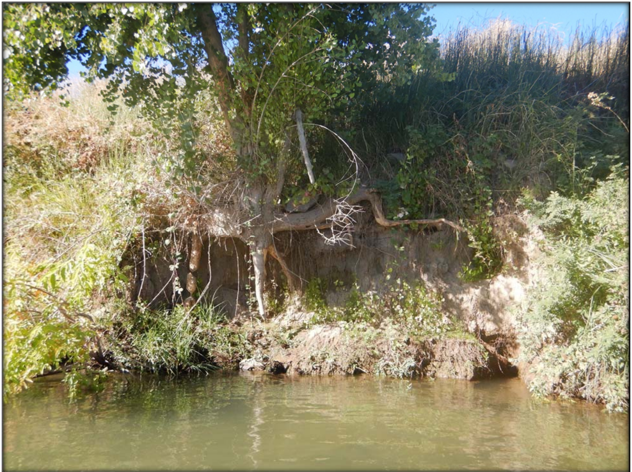
Figure 30. Scoured section of levee that has undermined a tree along the right bank of the Sacramento River at RM 38.5.
