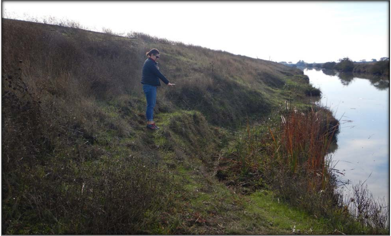
Figure 16. Slumps at Haas Slough LM 9.7 L.
