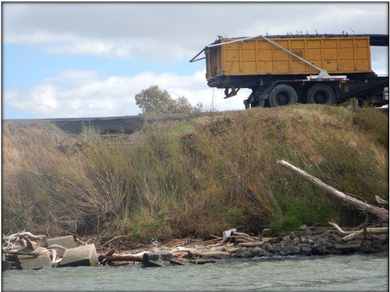
Figure 24 – Section of levee that has eroded under the highway along the left bank of the Sacramento River at RM 11.2.
