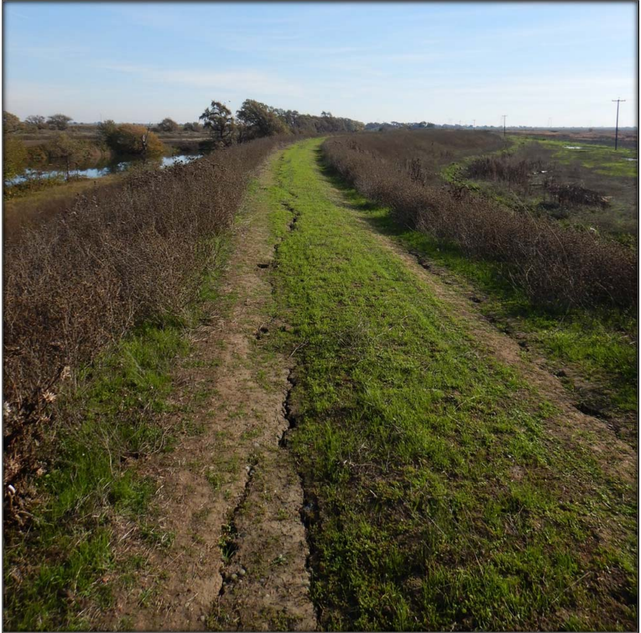
Figure 6. Slump Cracks observed on both the landside and waterside of Peters Pocket at Cache Slough, RM 1.8L.
