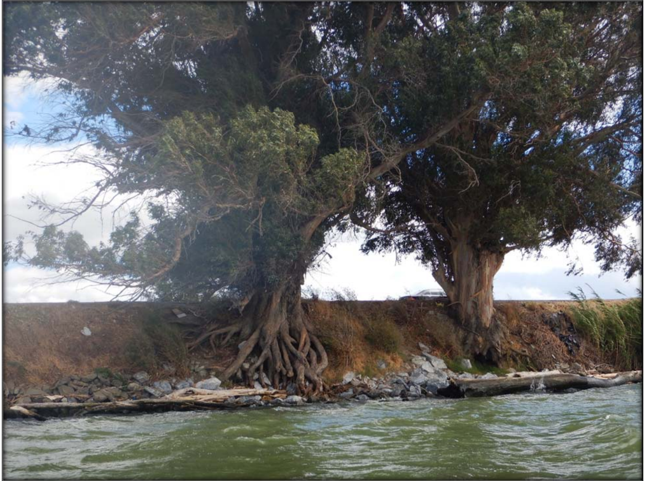
Figure 25. Eroded bank and large trees with exposed roots along the left levee slope of the Sacramento River at RM 11.2.
