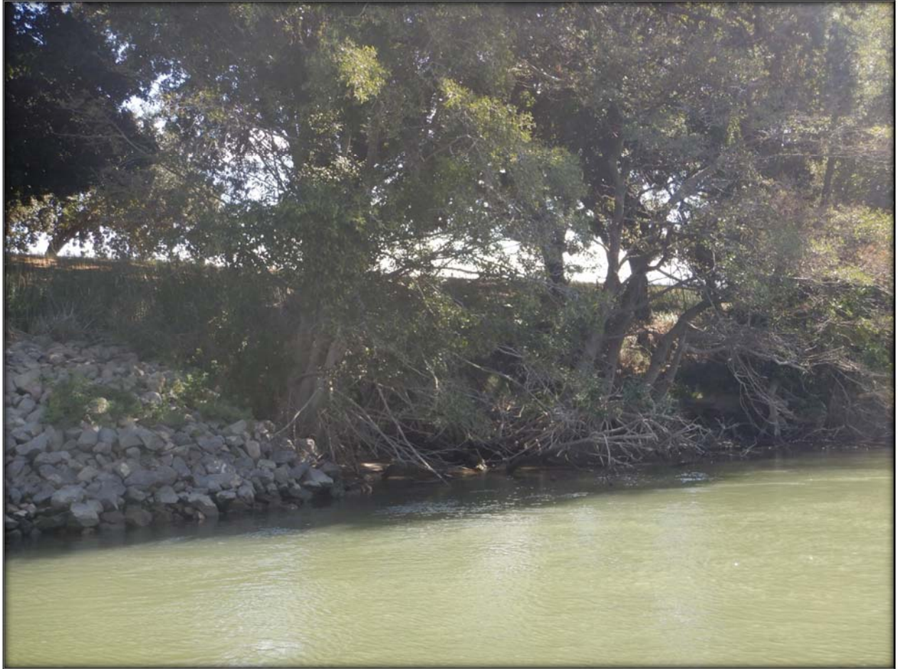
Figure 38. Eroded bank from eddy formation off adjacent rock protection along the left bank of Steamboat Slough at RM 25.0.
