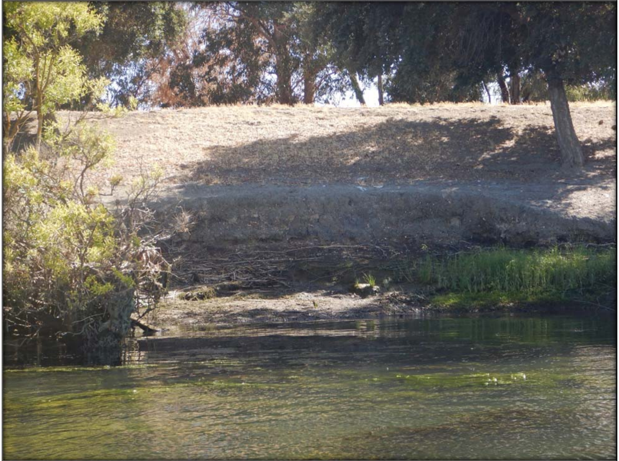
Figure 17. Erosion Pocket along the right bank of Lindsey Slough at river mile 0.7.
