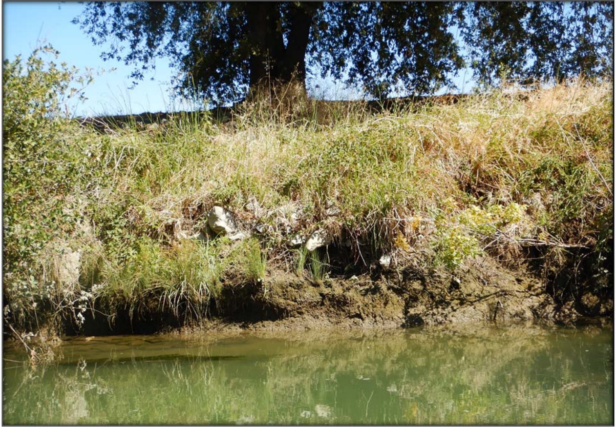
Figure 12. Typical toe erosion along the left bank of Georgiana Slough at river mile 9.3
