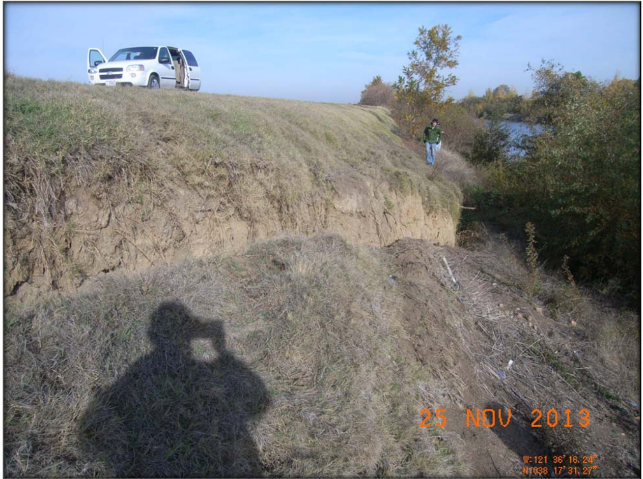
Figure 41. Large slump on the upper levee slope that occurred in 2013 along the right bank of Sutter Slough at RM 24.7.
