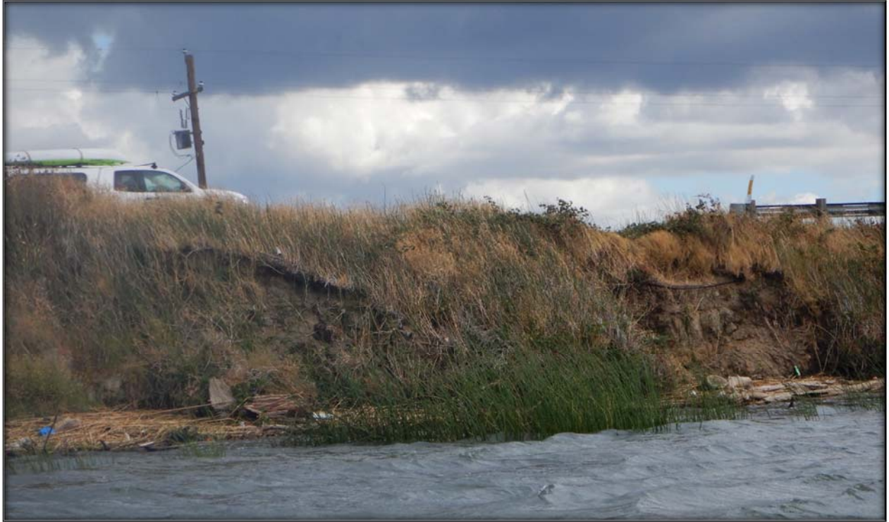
Figure 22. Bank erosion along the left levee slop of the Sacramento River at RM 8.0.
