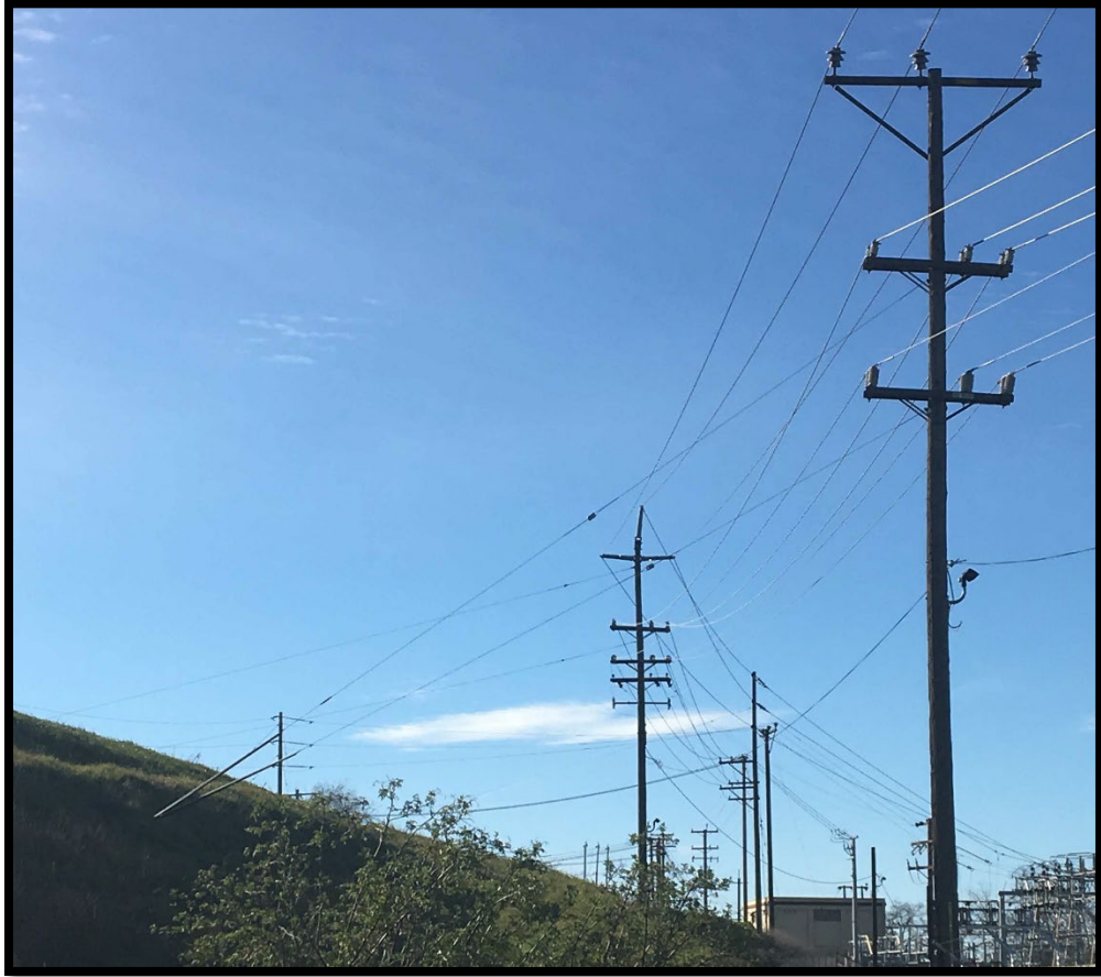
Figure 11. Guy Wire and Guy Wire Anchor Example.
