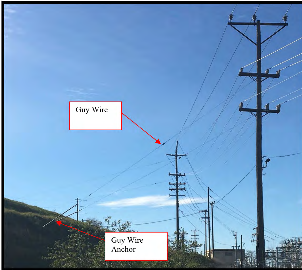
Figure 11. Guy Wire and Guy Wire Anchor Example.
