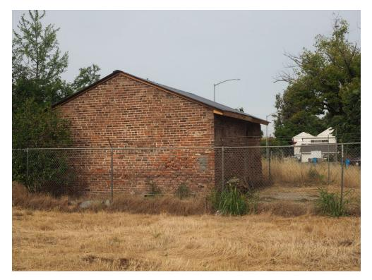
*Figure 7. Accessory building at 226 1st St., Marysville, CA. New roof added in 2018 now ties the walls together.*
