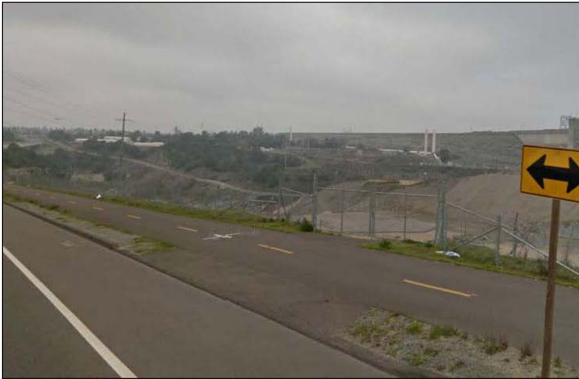
Figure 4. Access Road Entrance.
