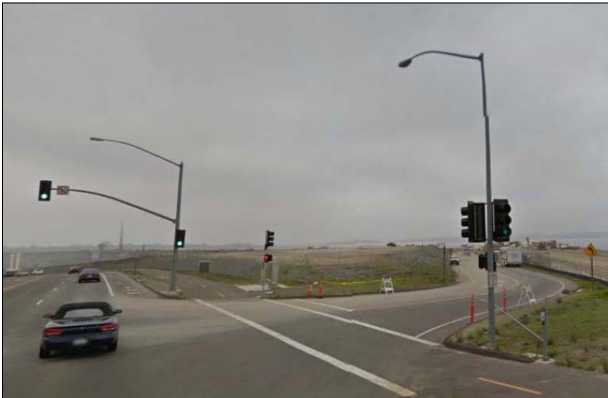
Figure 3. Intersection of Folsom Lake Crossing and Folsom Dam Road.
