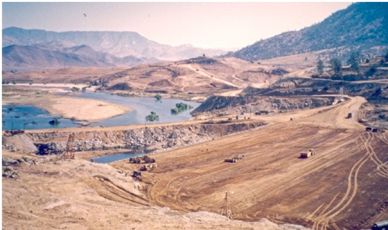
Isabella Dam construction site, c. 1950. Credit: San Joaquin Valley Library System.
