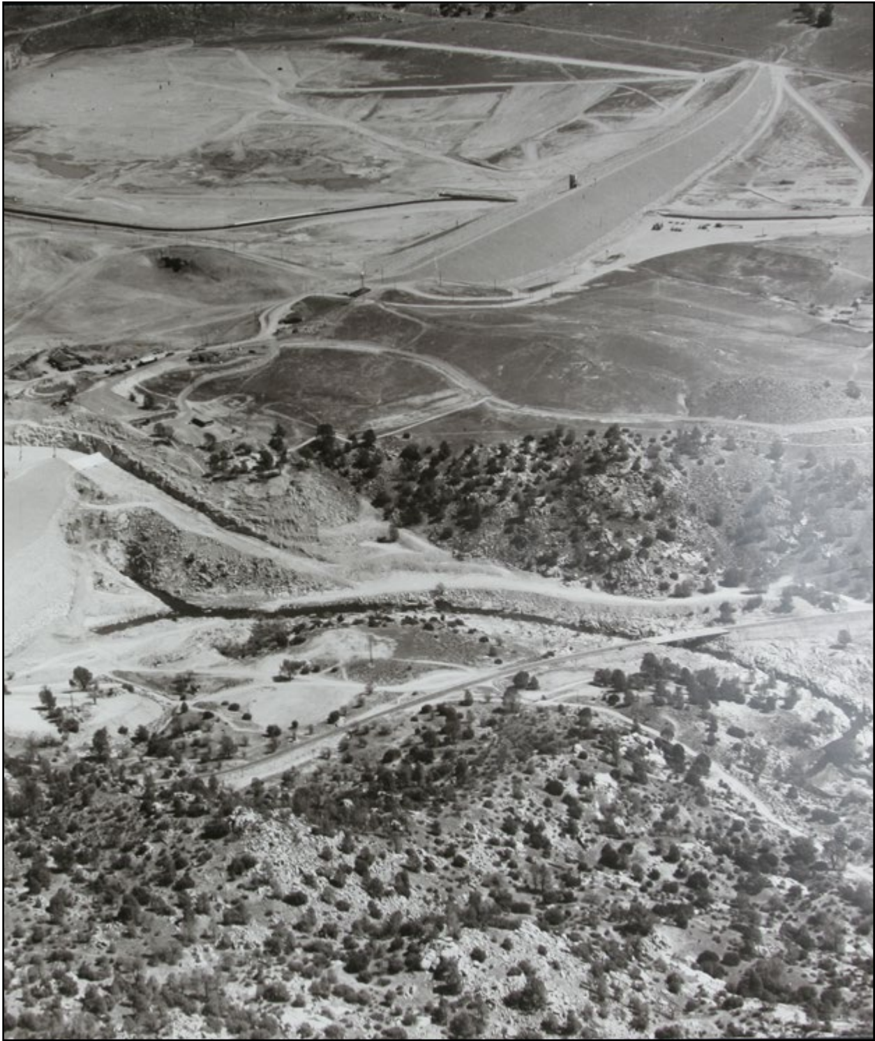
Aerial looking east at the completed Isabella Auxiliary Dam with empty reservoir, c. 1953.
