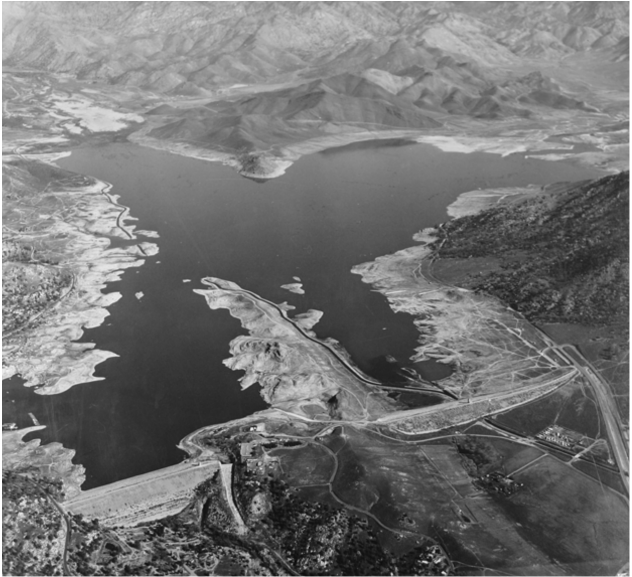
Aerial looking north at the Isabella Main Dam (left) and Auxiliary Dam (right), c. 1960.
