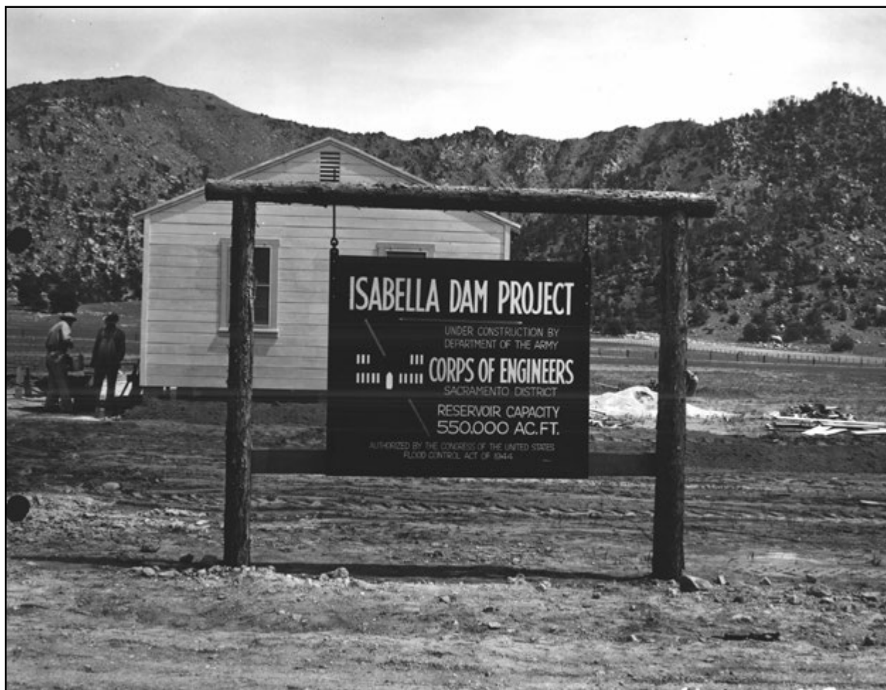
Isabella Dam project site, April 20, 1948.
