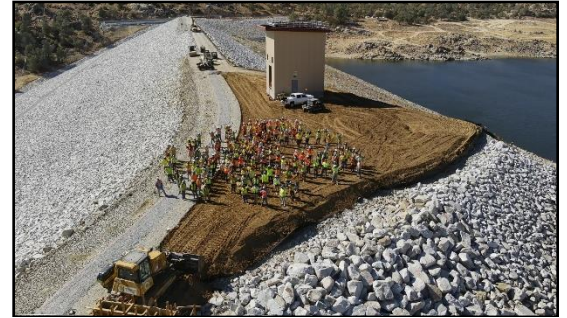
USACE and Contractor pose for a group photo at the Main Dam in celebration of top elevation core materials placement.
