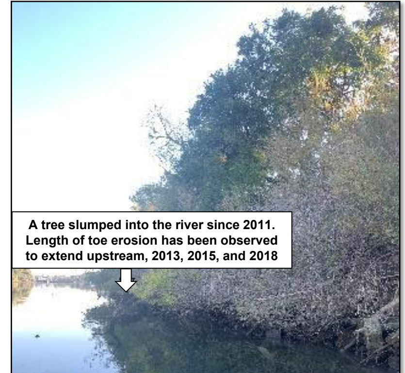
Survey on October 19, 2022 Photo taken looking upstream. Concrete placed along bank. Undercut below bank toe
