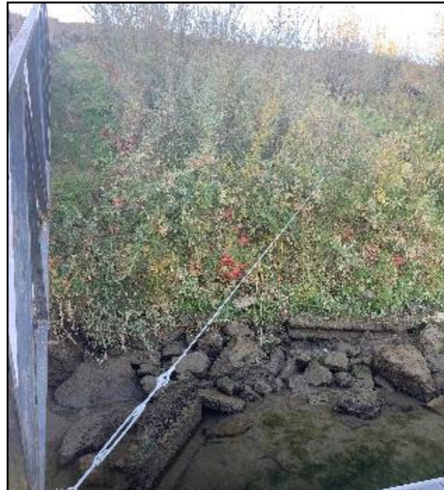
Survey on October 19, 2022 Photo taken looking up the bank slope. Concrete rubble placed at toe of bank. Willows growing above concrete.
