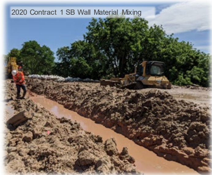
2020 Contract 1 SB Cutoff Wall Excavation
