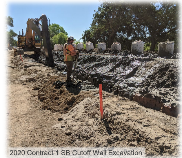
2020 Contract 1 SB Wall Material Mixing
