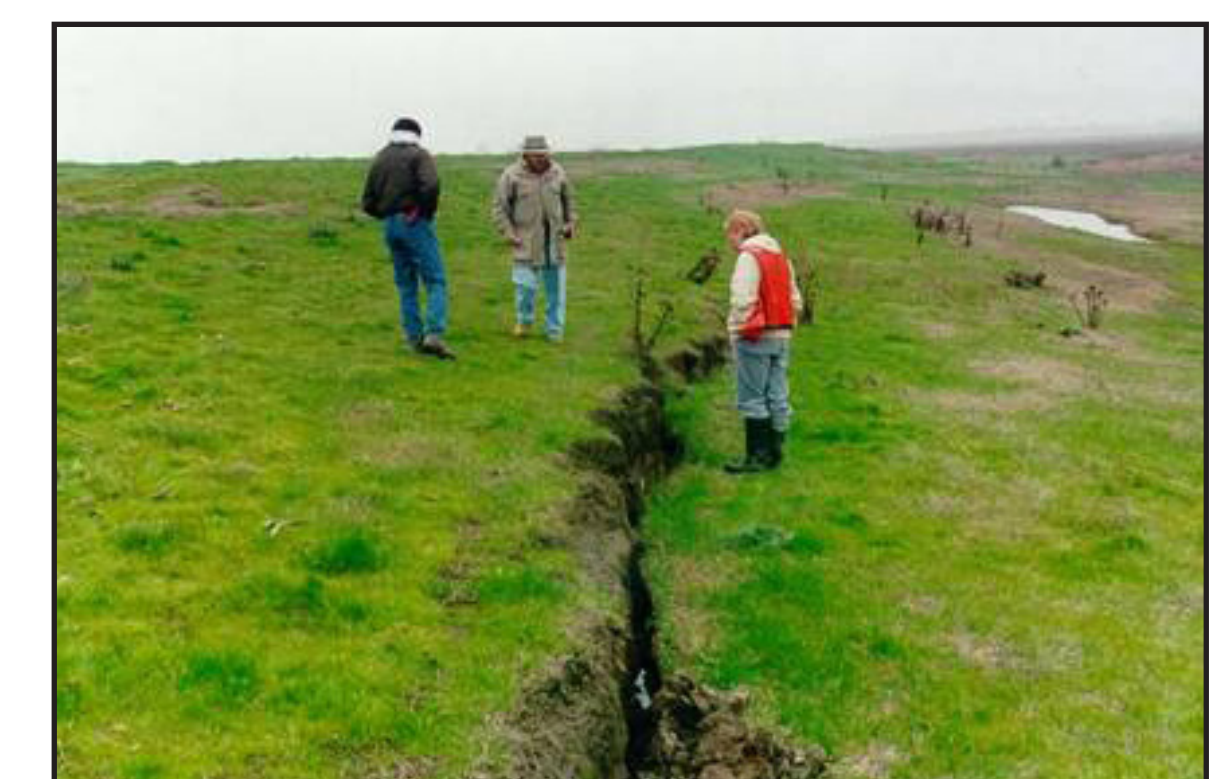
Levee instability problem
