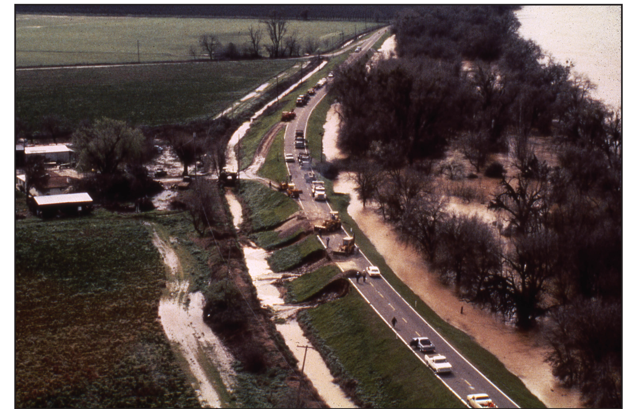
Seepage and stability problems
