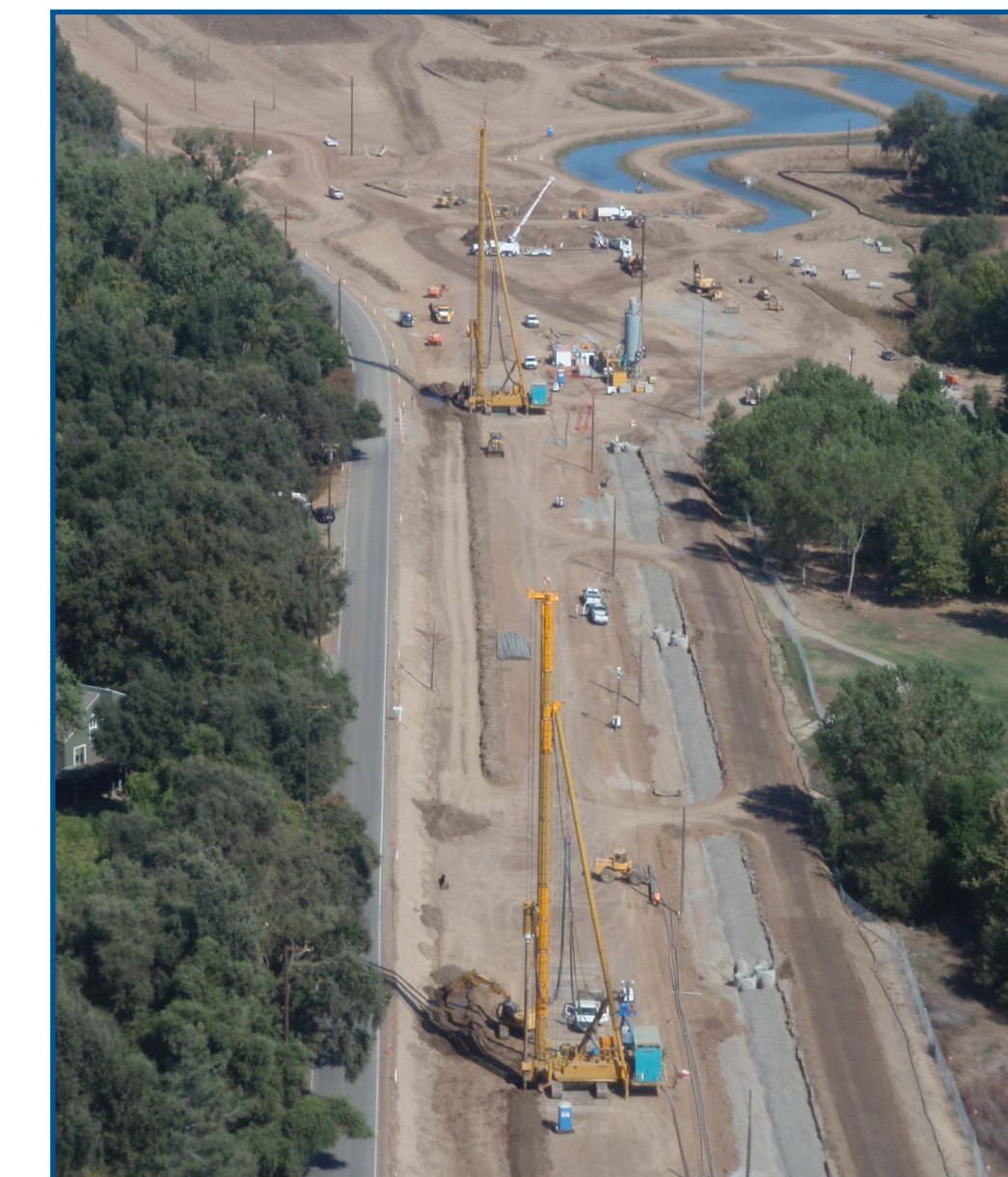
BELOW: Levee instability repair
