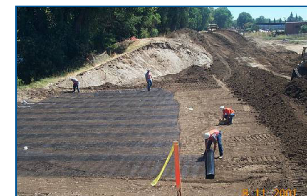
ABOVE: Levee instability repair
