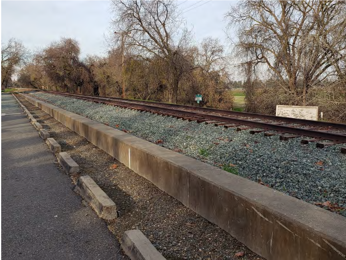
Figure 2-9. Existing flood wall at Cliff’s Marina on the SREL.
