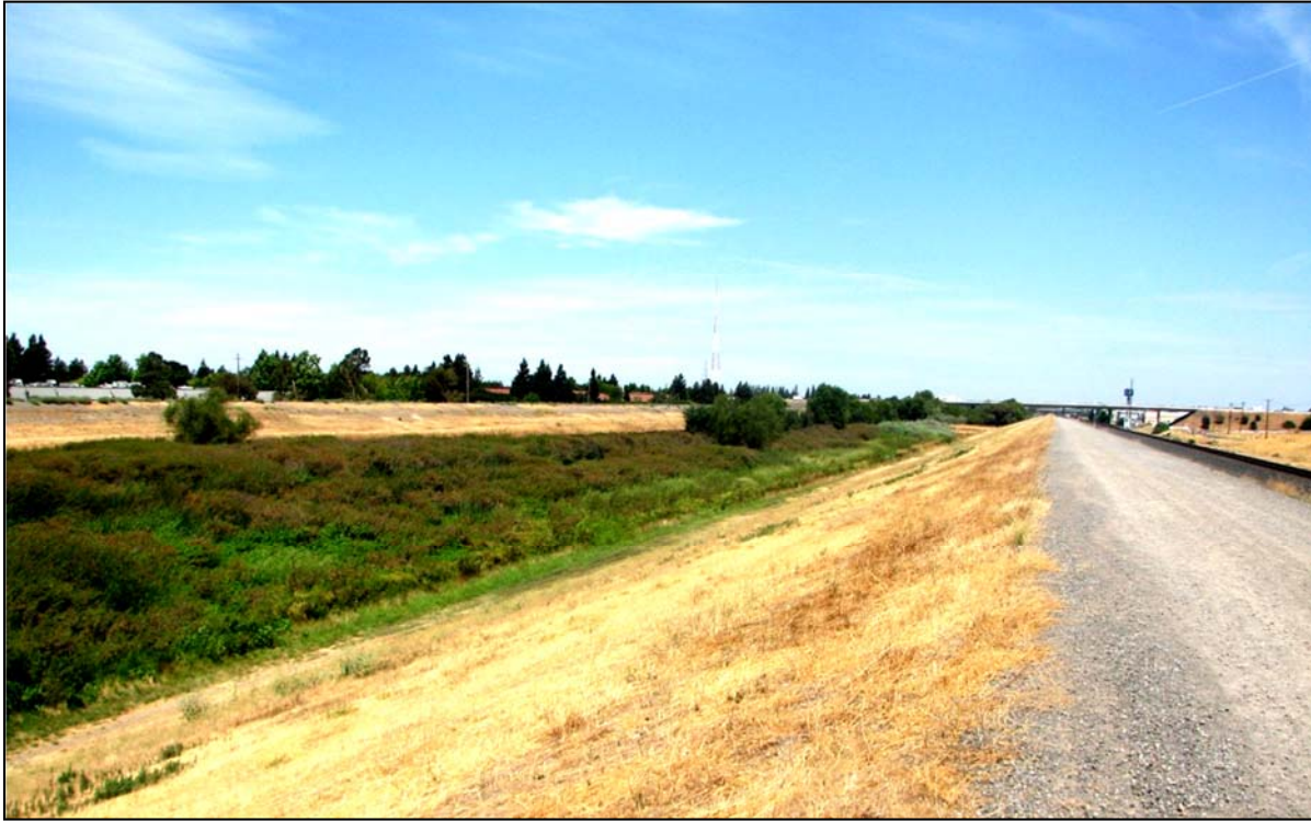
Figure 22. Natomas East Main Drain Canal.
