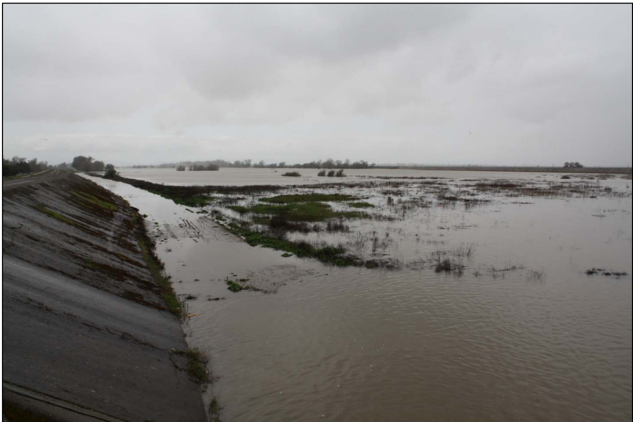
Figure 29. Sacramento Bypass (Downstream of Weir) with Water.
