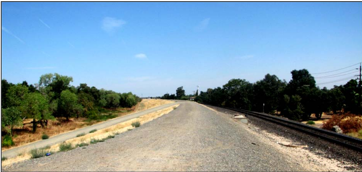
Figure 23. Natomas East Main Drain Canal Levee.
