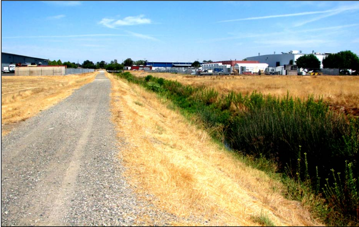
Figure 26. Magpie Creek Diversion Channel.
