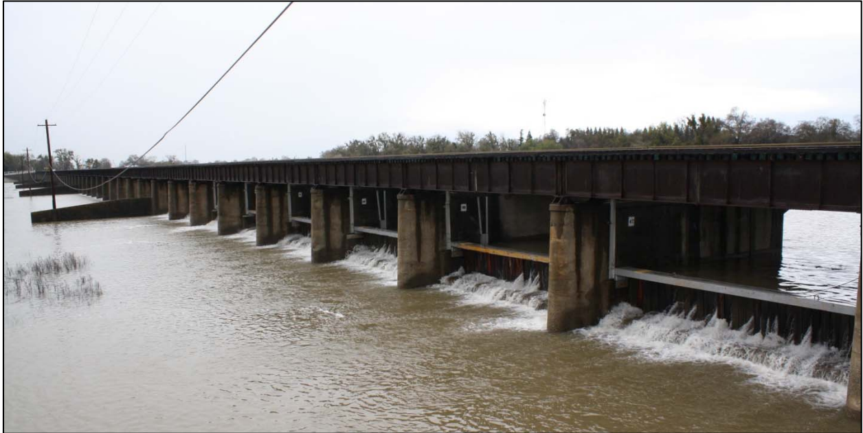
Figure 28. Sacramento Weir in High Water Event.
