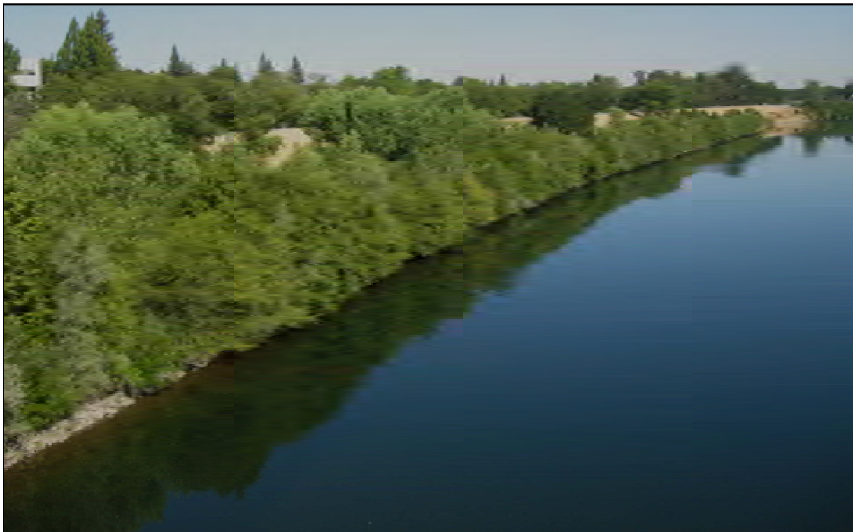
Figure 24. Bank Protection Site 4R in 2010.
