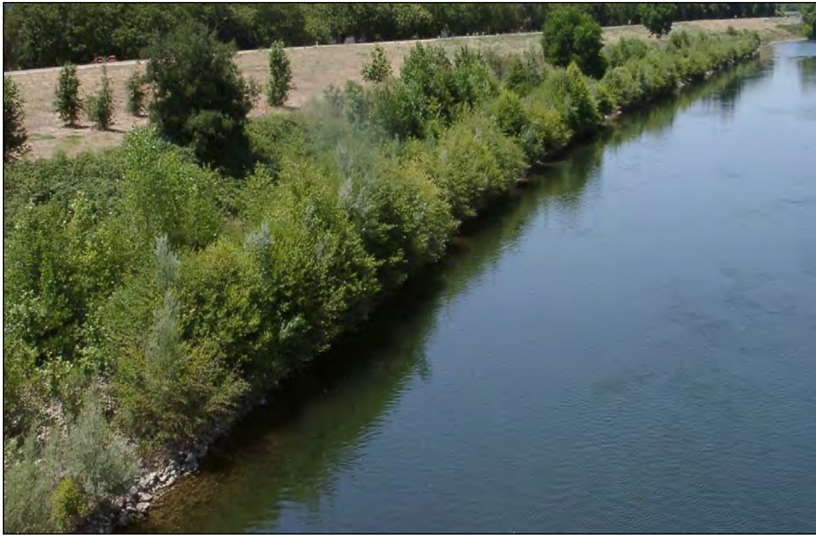
Figure 23. Bank Protection Site 4R in 2005
