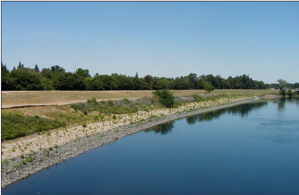
Figure 22. Bank Protection Site R4 in Planting Year 2001 on the American River.
