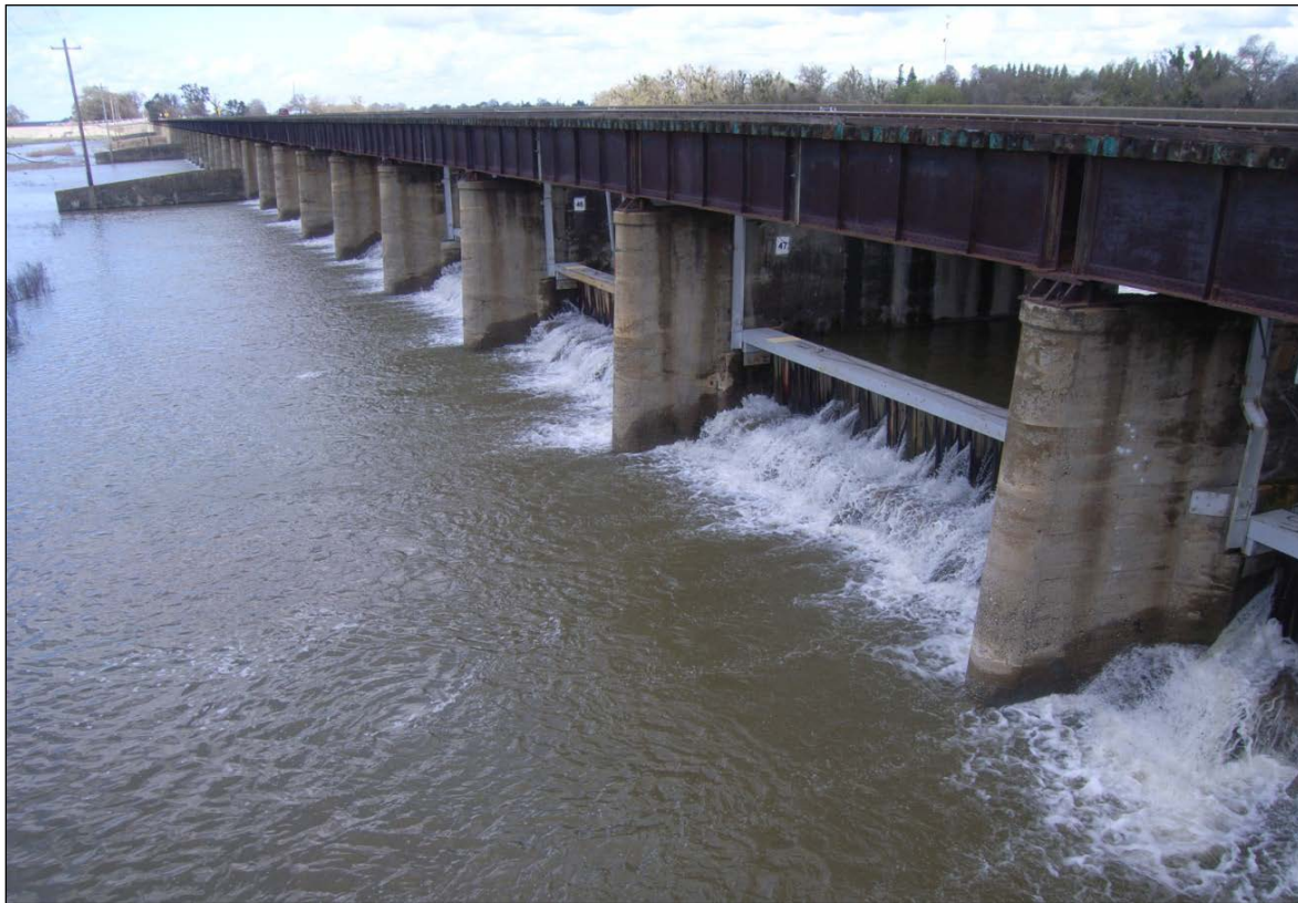
Figure 1-8: The Sacramento Weir.
