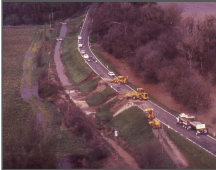
Figure 2-1: Slope Failures on the Landslide of the Levee and Seepage Exiting at the Levee Toe on the Garden Highway in Natomas during the 1986 Flood.
