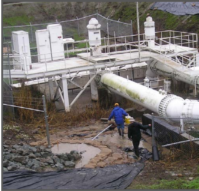
Figure 2-3: Sandbag Ring Surrounds a Sand Boil on the Natomas Levee during the 2006 Flood.
