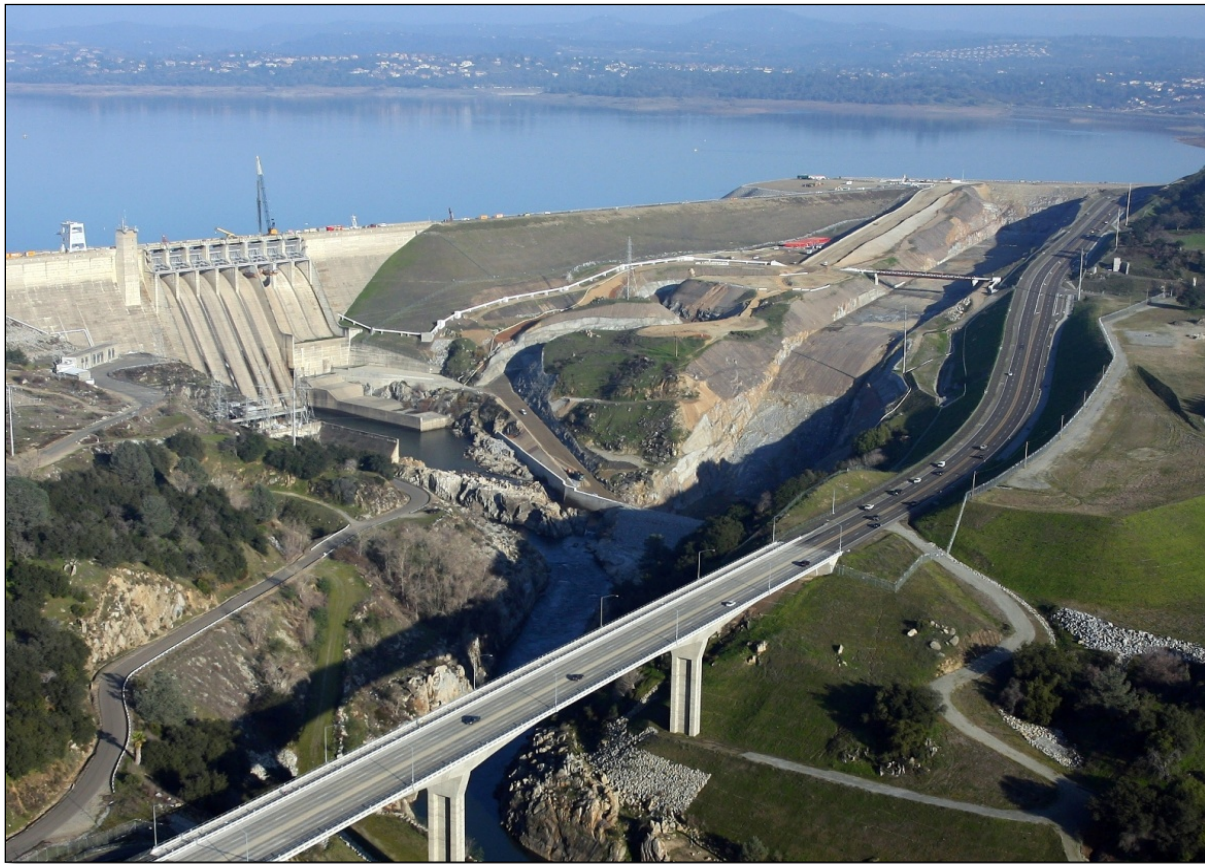
Figure 2-10: Construction in Progress at Folsom Dam as part of the Folsom JFP.
