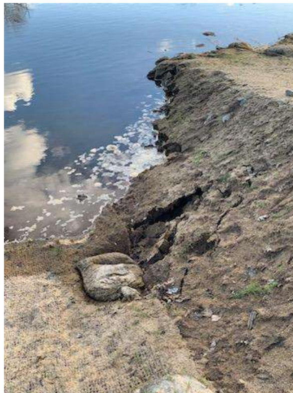
Figure 38: Eroding Tieback and Planting Bench
