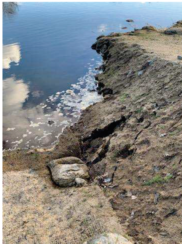
Figure 38: Eroding Tieback and Planting Bench
