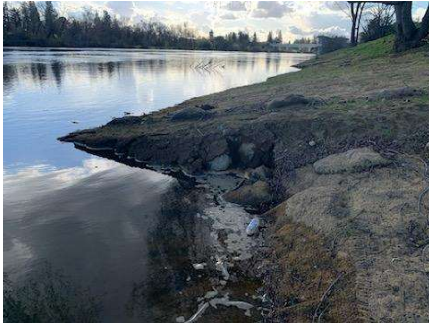
Figure 37: Eroding planting bench and tieback with the riprap already exposed.
