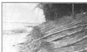
FIG. 3—MISSISSIPPI RIVER PROJECT Willow Poles 40-ft. Long in Position to be Protected With Branch, Stakes and Wire Fencing
