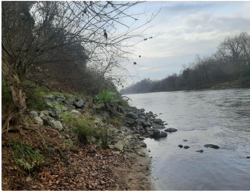
Figure 41: Riprap at left bank river mile 10.3-10.4
