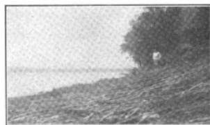
FIG. 4—MISSISSIPPI RIVER PROJECT Brush Mattress for Protection of Willow Poles and Bank
