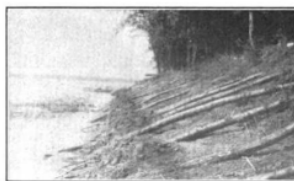
FIG. 3—MISSISSIPPI RIVER PROJECT Willow Poles 40 ft. Long in Position to be Protected With Brush, Stones and Wire Fencing
