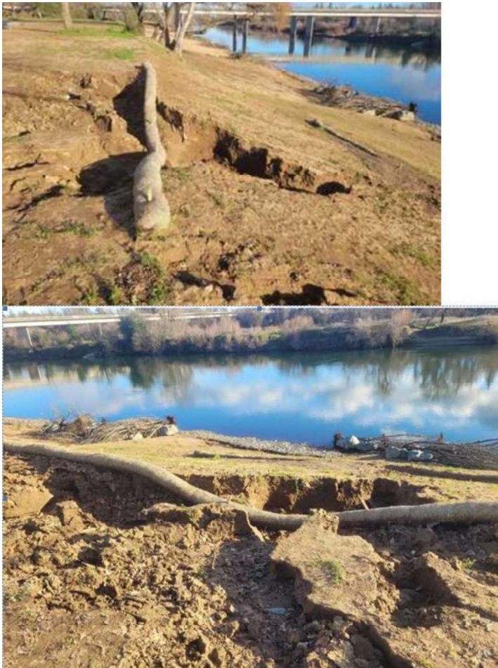
Photo of new Contract 2 soil surface being rapidly washed away by rain and river waves. Again, this level of erosion is never seen in a natural intact bank.
