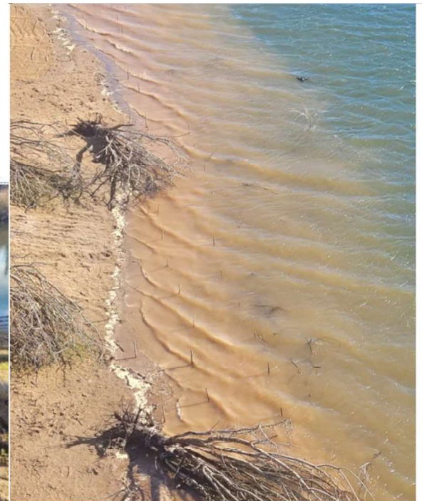
Photo of new Contract 2 soil surface being rapidly washed away by rain and river waves. Again, this level of erosion is never seen in a natural intact bank.
