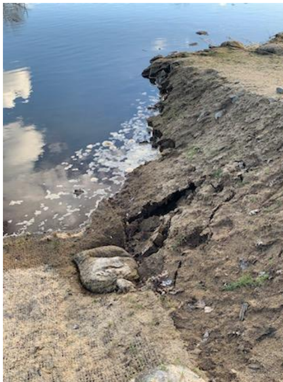
Figure 38: Eroding Tieback and Planting Bench
