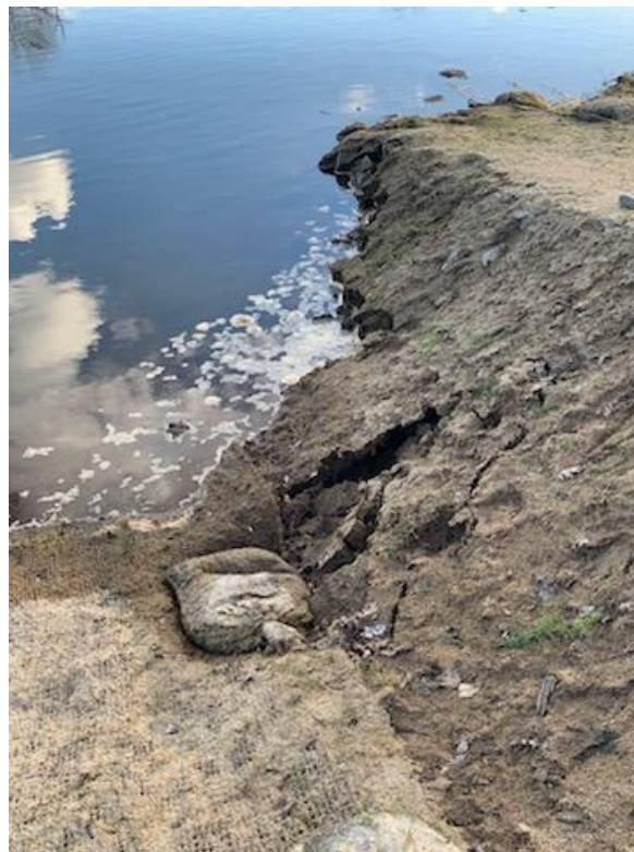
Figure 38: Eroding Tieback and Planting Bench
