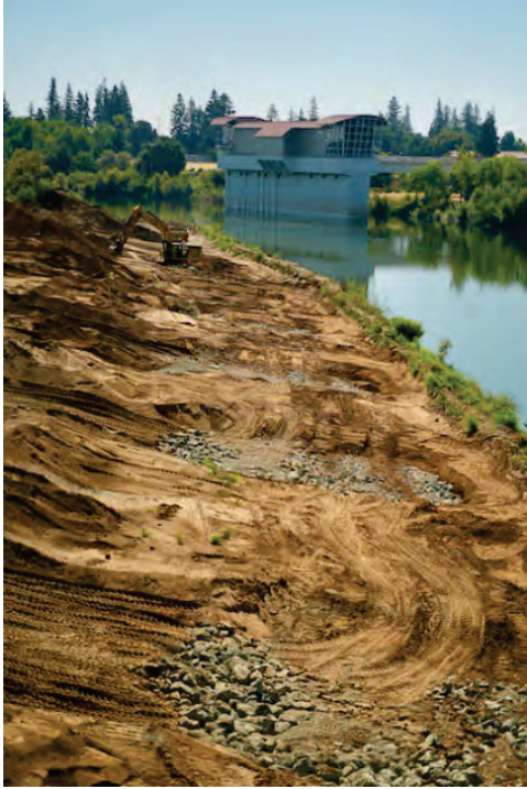
Figure 5 - Looking upstream from Guy West Bridge, 8/26/2023, installation of riprap/revetment
