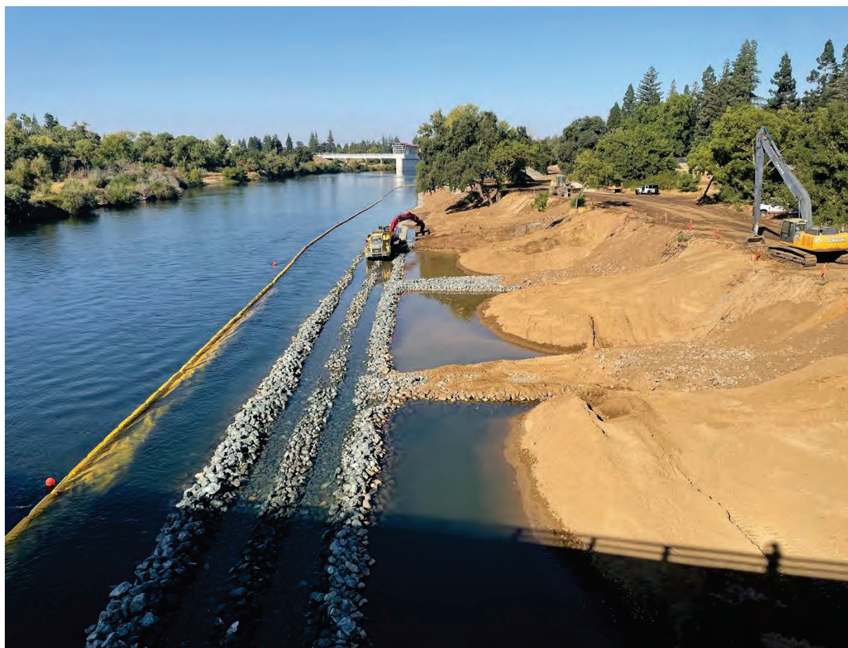
Figure 16 – Launchable toe, proposed for Project area, applied downstream of Project area
