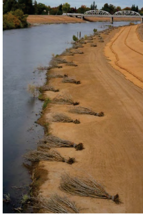
Figure 6 - Looking upstream from Guy West Bridge, 11/5/2023, revegetation phase on buried riprap
