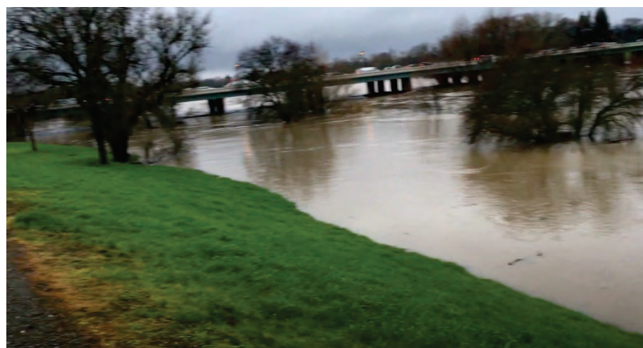
Figure 21 - Watt Bridge area near time of peak flow in Water Year 2017 (~80 kcfs shown), nearing "bank full" conditions, with slow moving/backwater conditions at the levee. Roughly twice as much flow would need to pass through here in a 200 yr storm event given the new 160 kcfs limit chosen for control of a 200-yr event
