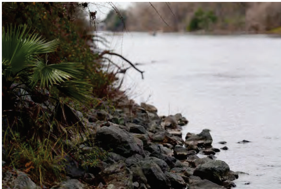
Figure 92 - LAR riverbank post ARCF project, with soil eroded away from riprap (RM ~10.3) (WY 2024)
