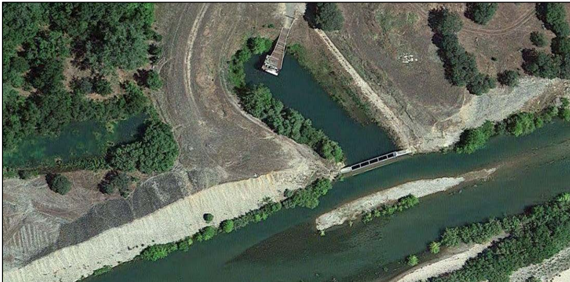
Figure VIII-13. BVID diversion facility, including the fish screen and diversion forebay (Source: YCWA 2013b).
