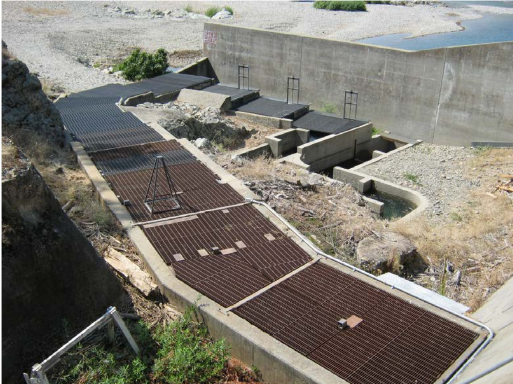
Figure IV-3. South fish ladders at Daguerre Point Dam (Corps 2013b).
