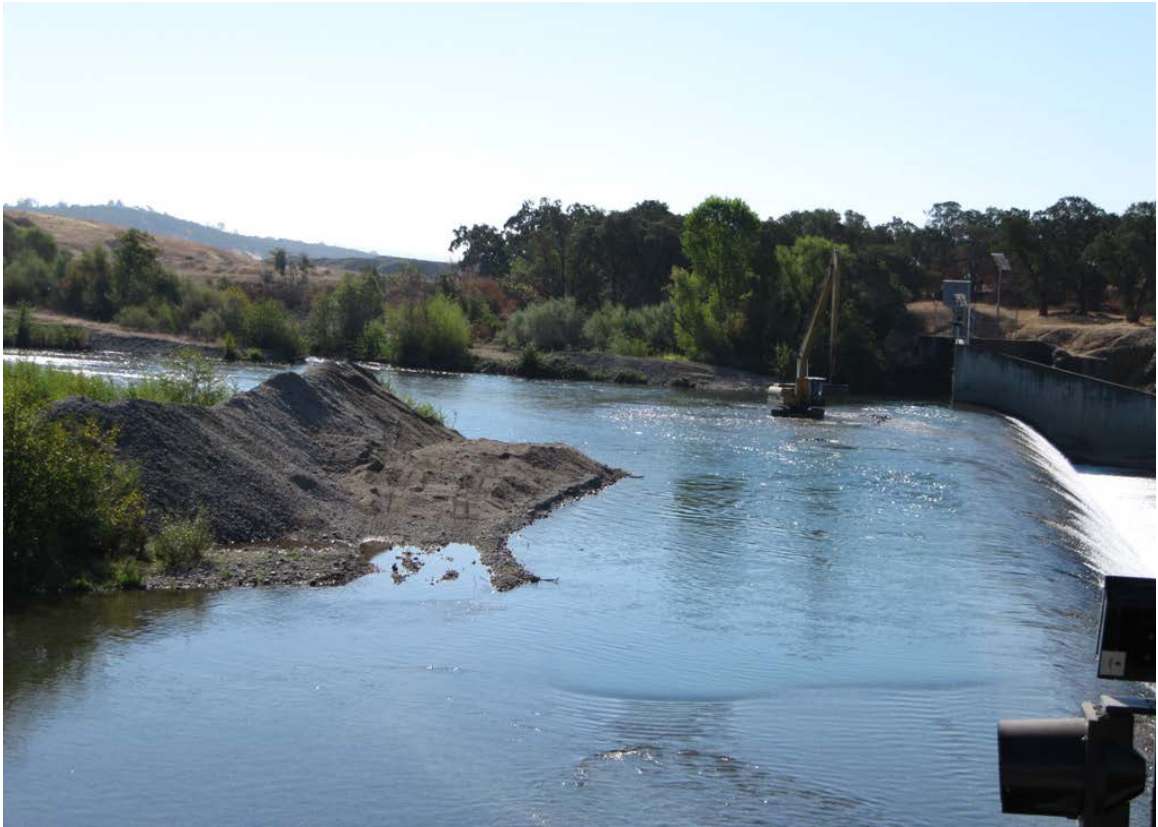
Figure IV-4. Excavator removing sediment above Daguerre Point Dam during August 2011.
