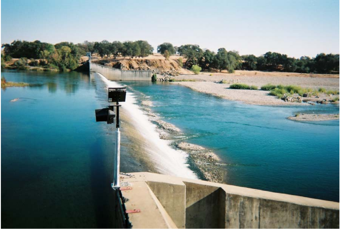
Figure IV-1. Daguerre Point Dam (photo by D. Simodynes, October 9, 2009).
