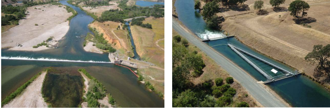
Figure VIII-10. Hallwood-Cordova Diversion. Image on the left shows the control gate headworks on the north abutment of Daguerre Point Dam. Image on the right shows the current v-shaped screen (Source: YCWA 2013b).
