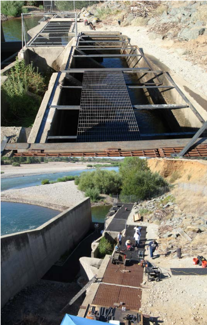
Figure VIII-6. Installation of metal grates on the Daguerre Point Dam fish ladder bays during August 2011 (Corps 2011).
