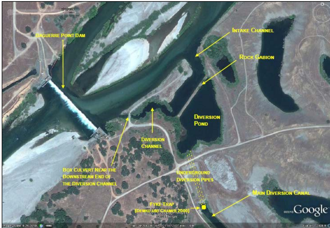
Figure VIII-11. Diversion headworks area for the South Yuba/Brophy Diversion Canal and Facilities.
