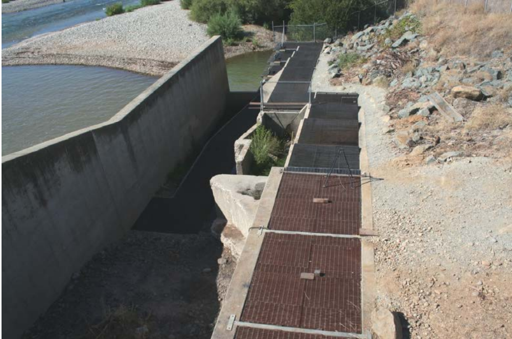
Figure IV-2. North fish ladders at Daguerre Point Dam (Corps 2013b).
