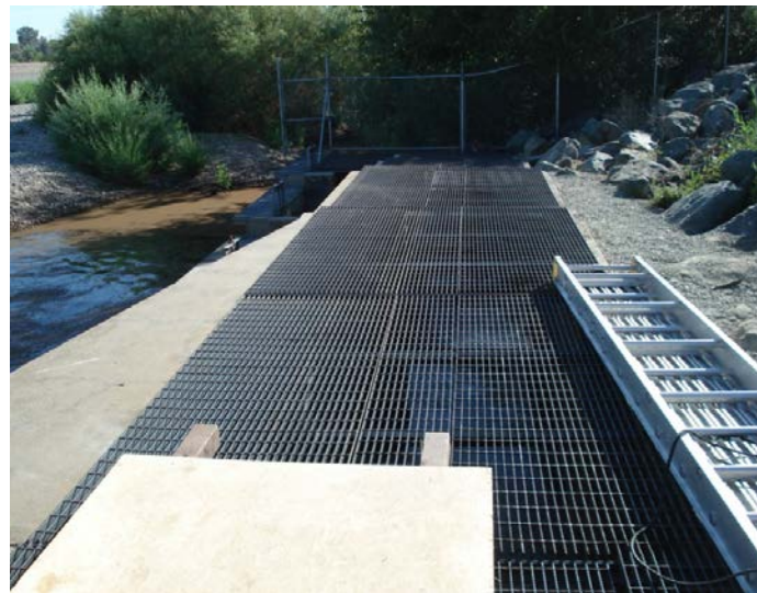
Figure VIII-6. Installation of metal grates on the Daguerre Point Dam fish ladder bays during August 2011 (Corps 2011).
