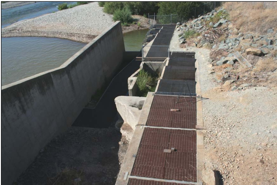
Figure VIII-7. North fish ladders at Daguerre Point Dam (Corps 2012c).
