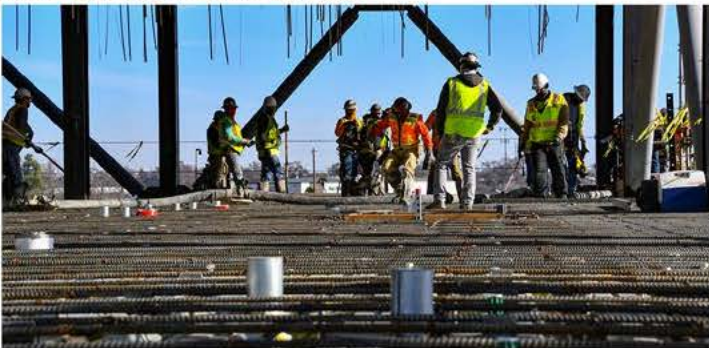
Floor construction January 2021
