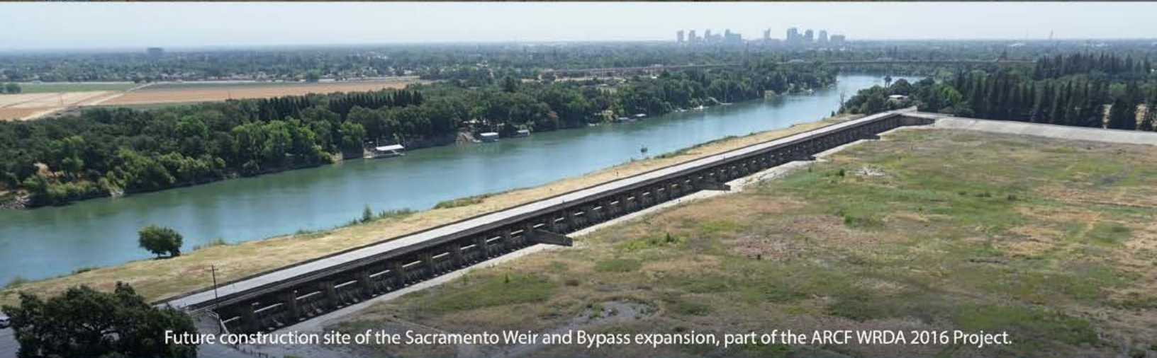
Completed construction on Dike 8, part of the Folsom Dam Raise Project, Folsom, Calif.
