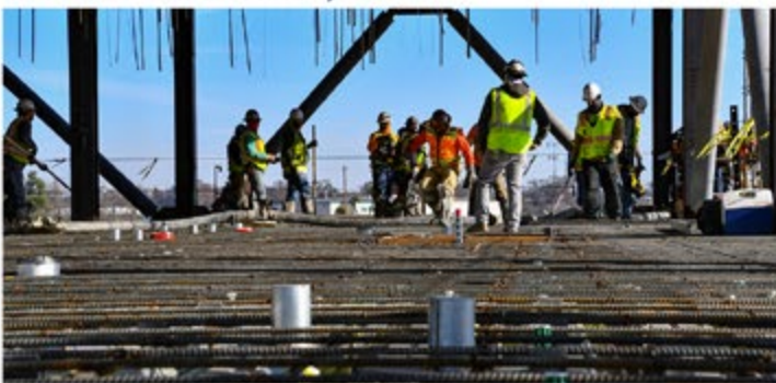
Floor construction January 2021
