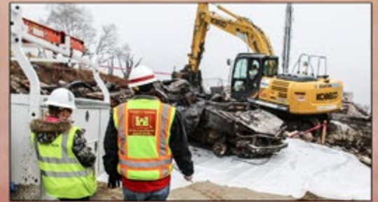
Corps' contractors remove debris in Lake County, California, Jan. 7, 2018. Photo by Carol Vernon.
