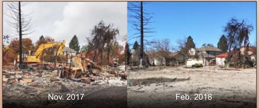
A before and after comparison of debris removal shows progress on a property in Santa Rosa, California. Final steps on many properties will include hydro-seeding, final inspection and clearance for the owner to rebuild. Photos by Rick Brown.
