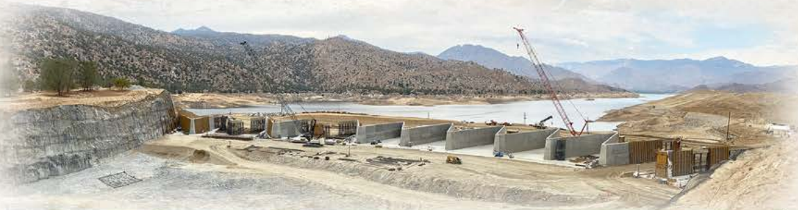
New construction work on the Isabella Dam Safety Modification Project, Aug. 12, 2021. The project will reduce the risk of catastrophic floods resulting from dam breach for downstream communities. Credit: John Prettyman
