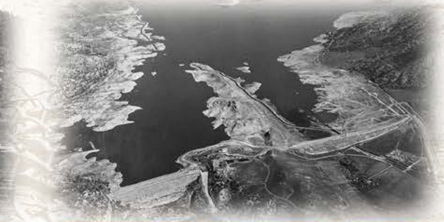
The completed Isabella Main Dam (left) and Auxiliary Dam (right), c. 1960.
