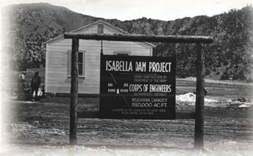
Isabella Dam project site, April 20, 1948.
