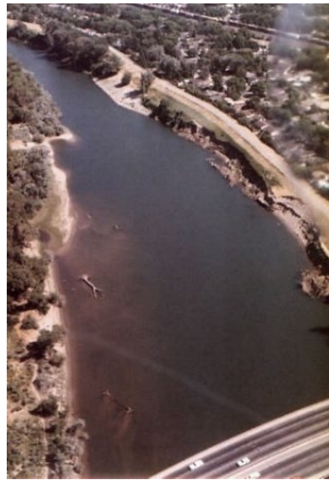
River Park neighborhood adjacent to I-80 bridge 1986 Levee erosional event
