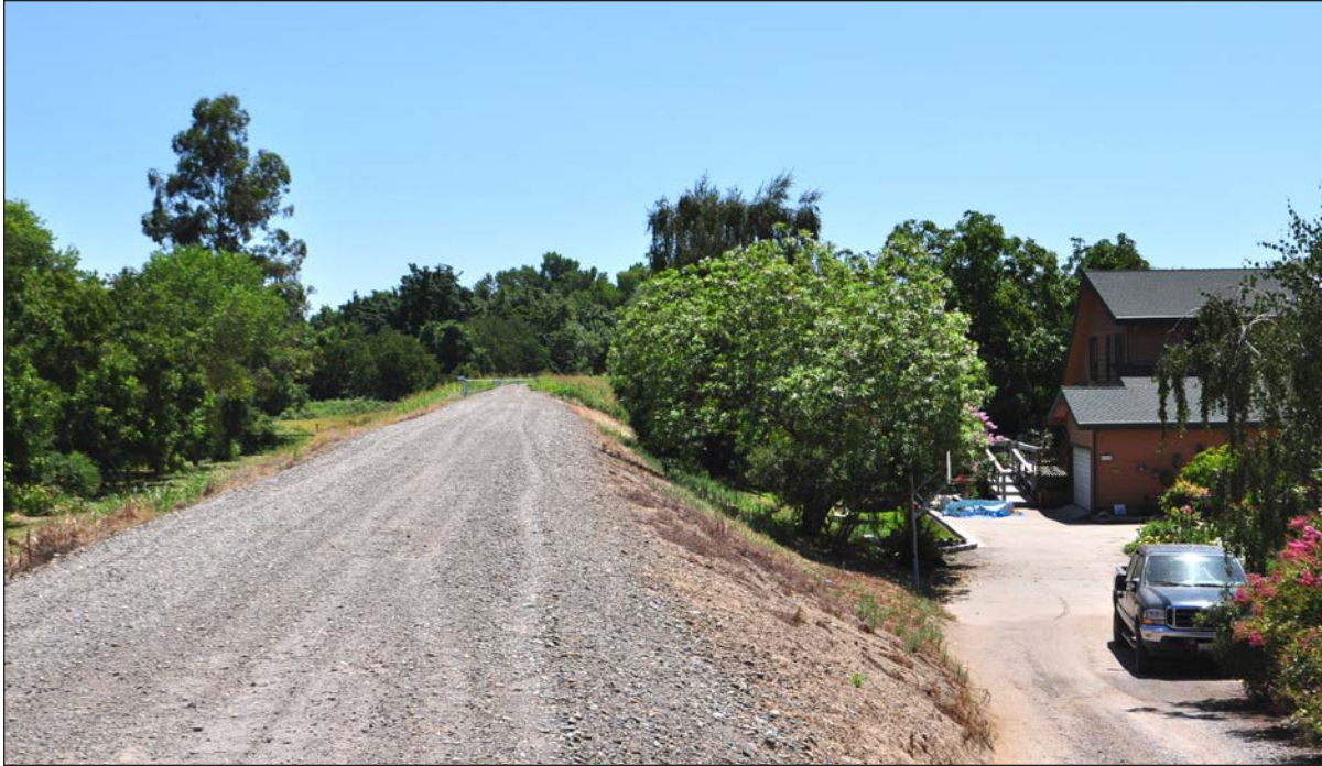
Reach 23. Feather River west levee looking south from the levee crown. Note the residence on the landside toe and the mature vegetation on both the land and watersides of the levee.
