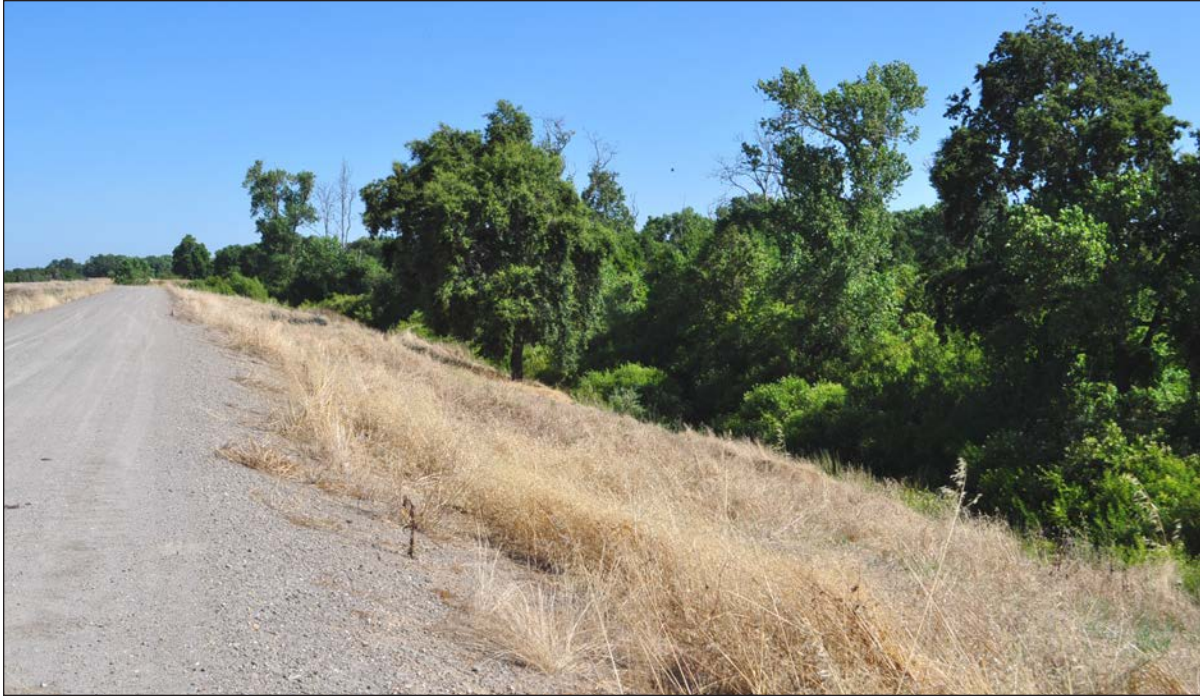
Reach 4. Feather River west levee looking northeast from water side of levee crown. Note mature vegetation on waterside slope. River is off the photo to the right.
