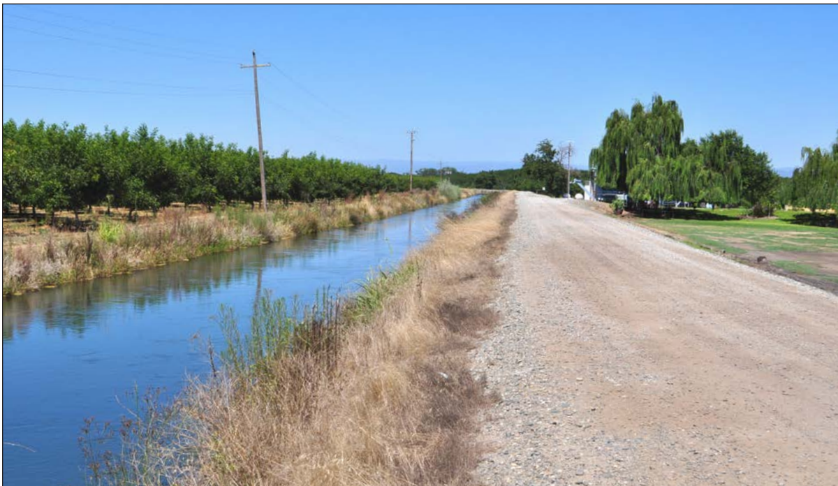
Reach 26. Feather River west levee looking north from land side of the crown. Note the irrigation canal, utility poles, and orchards to the left. Also note the decreased levee prism in this reach.
