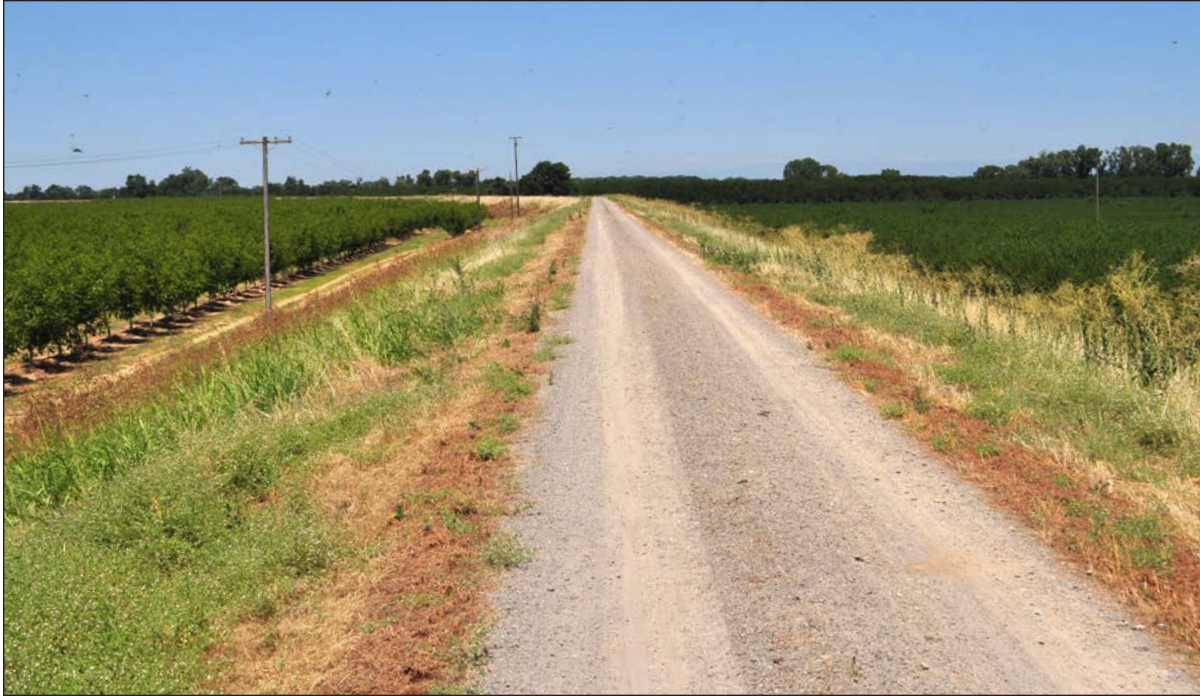
Reach 18. Feather River west levee looking north from the levee crown. Note the utility poles at the landside toe of the levee at left with orchards beyond.
