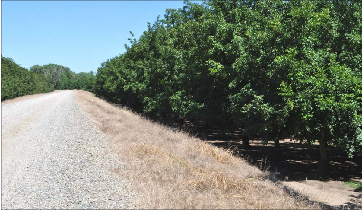
Reach 32. Feather River West levee looking north from the water side of the levee crown. Note orchards on both water side and land side of the levee.
