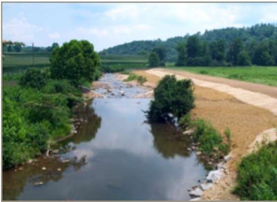
Figure 9.1a Restoration site immediately after construction.
