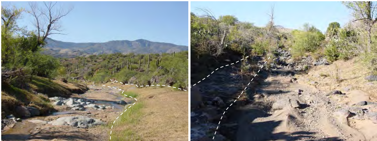
Figure 23. Examples of narrow berms below the OHWM along channels in central Arizona. In each case, the berm lies below the upper dotted line , which approximates the OHWM, and the lower dotted line .
