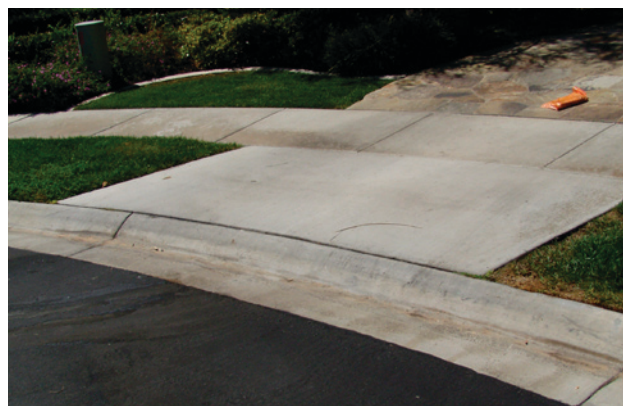
Typical Rolled Curb
