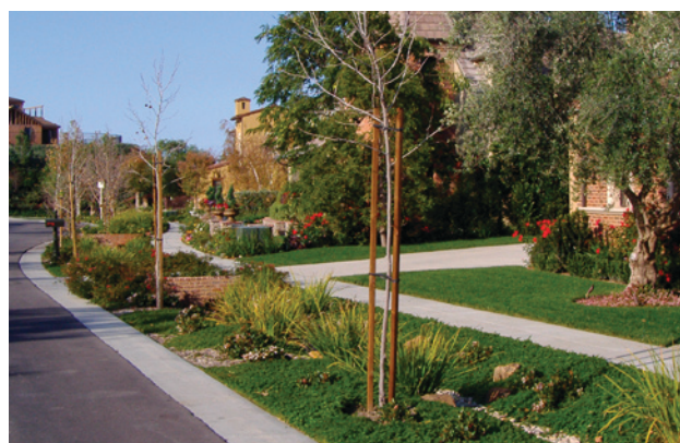
Typical Rolled Curb at a Bioswale
