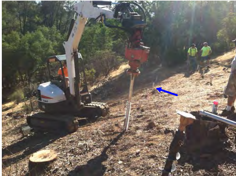
Example of a crawler driving “earth screws” into a steep slope to serve as the foundation for solar racking. The blue arrow shows previously driven screws. Moving material and equipment is more time consuming than equivalent work on level land.
