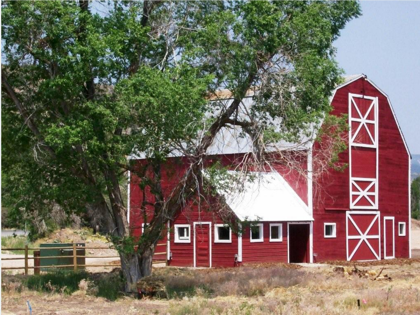
Building restoration, Victory Ranch, near Kamas, UT
