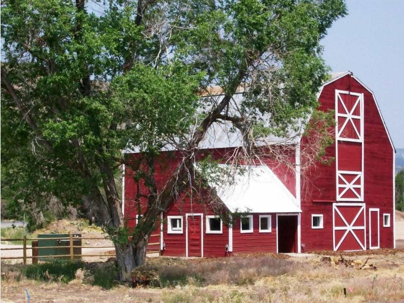
Building restoration, Victory Ranch, near Kamas, UT (courtesy of Jeff Graham)
