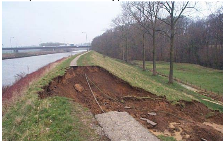
Figure 6. Sloughing of levee slope as a result of stability problem
