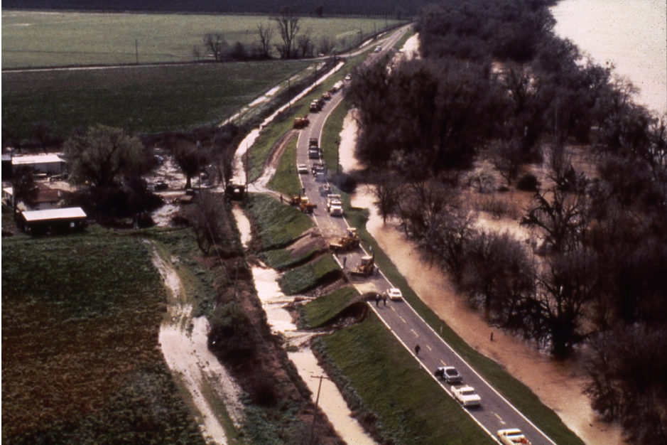
Figure 1. Seepage and stability distress in Natomas during the 1986 flood event
