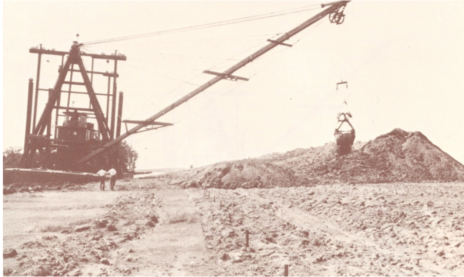
Figure 3. Typical clamshell dredge levee construction on the Sacramento River system
