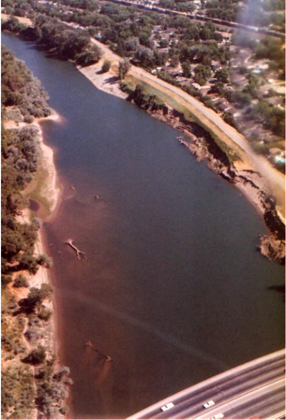
Figure 2. Erosion distress on the American River after the 1986 flood event
