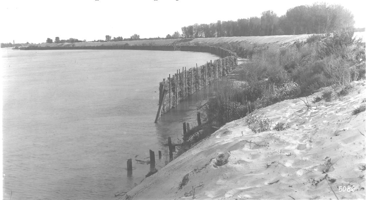
Figure 3-5: Levee Constructed Near Davis Road, West Sacramento
