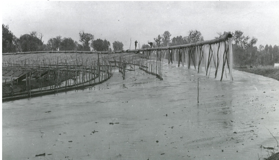
Figure 4. Typical suction dredge levee construction on the Sacramento River system
