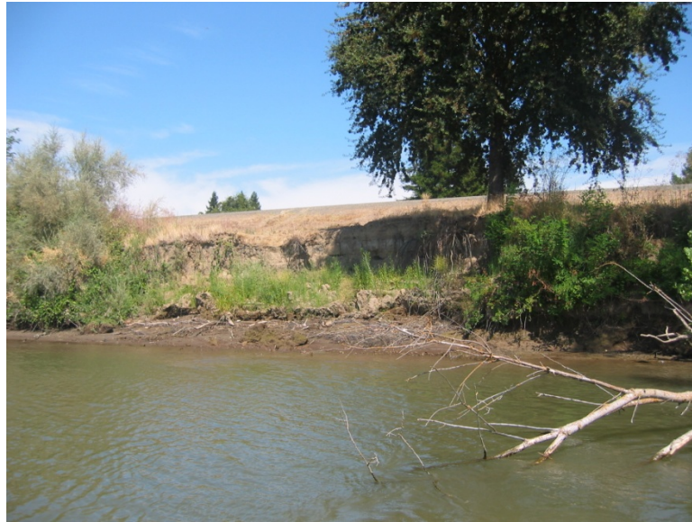
Figure 7. Erosion of the levee slope on the Sacramento River.
